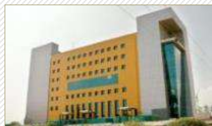
Airtel Data Center - Chennai
