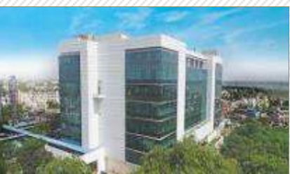
TATA Data Center - Chennai
