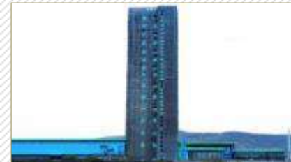
121m Tall VCV Tower - Pune
