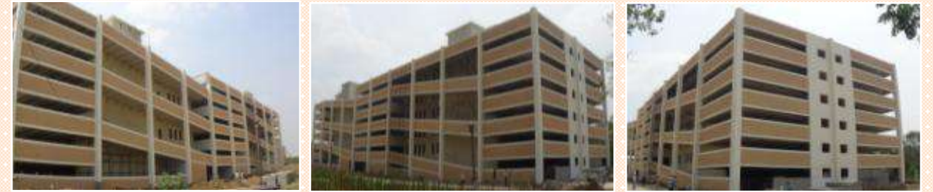
Precast Multi-Level Vehicle Parking Building (G+5) for M/s Infosys at Chennai
