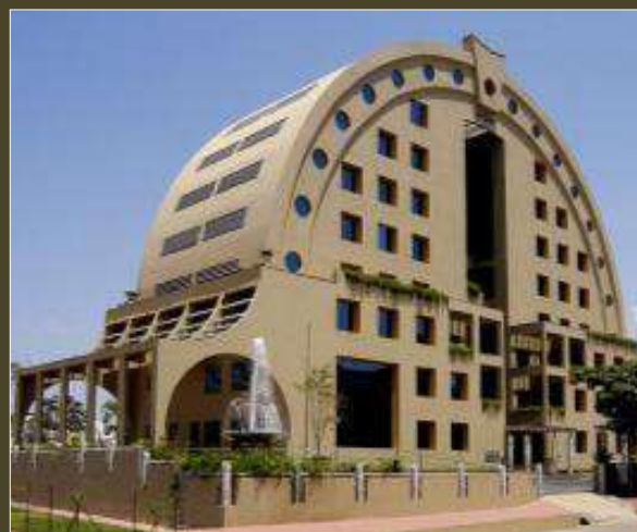
Office Building (Jal Bhavan) for Karnataka Water Supply & Sewerage Board in Bangalore
