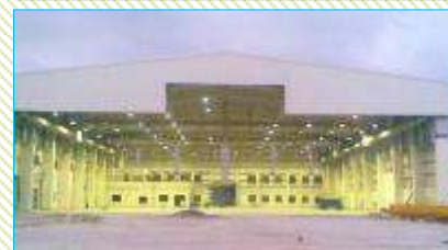
Hangar Building, Trivandrum
