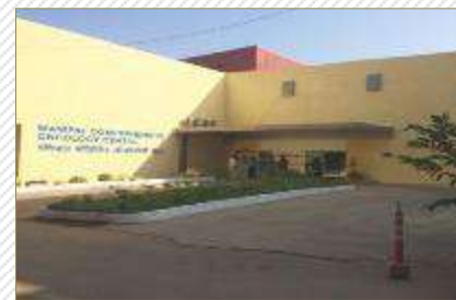
ManipalLinac Hospital - Goa
