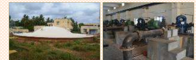
Clear Water Sump
