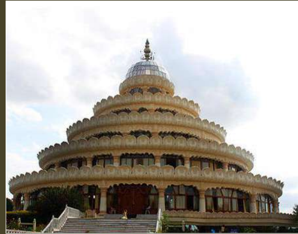
Vishalakshi Mantap - Meditation Hall for Art of Living International Centre in Bangalore
