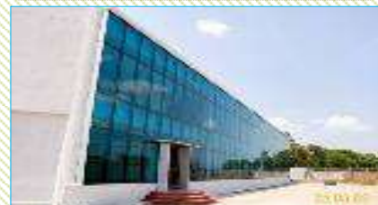
Line Maintenance Building, Chennai
