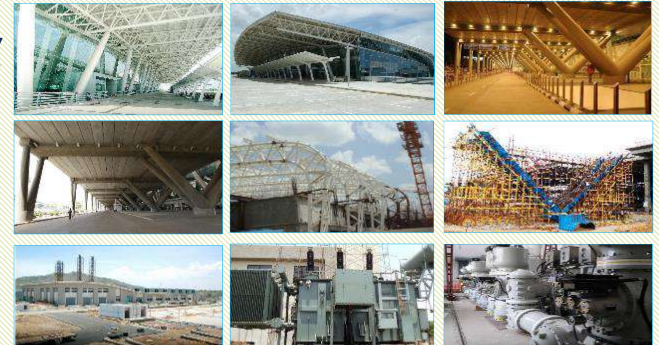
110KVA Gas Insulated Switchgear(GIS) Substation
