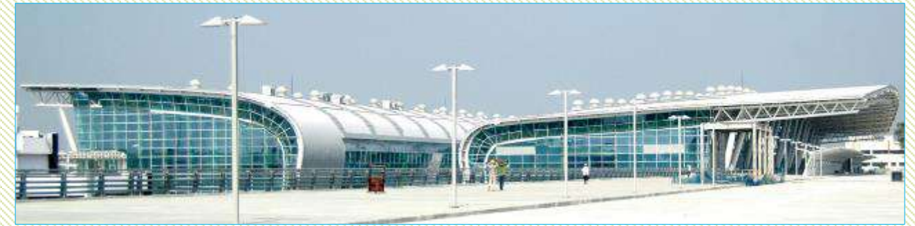
It's all about Chennai Airport – Phase I Construction
