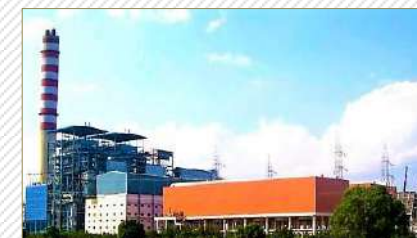
IND Bharath Power Plant
