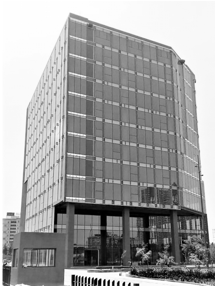
South West Multi-use Retail (SWMR) -Commercial Building for M/s Karle Infra Pvt Ltd at Bengaluru, Karnataka.
