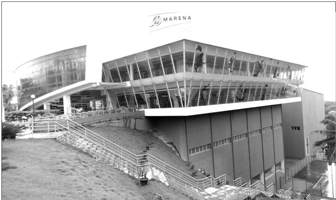
Manipal Sports Complex Building, Manipal
