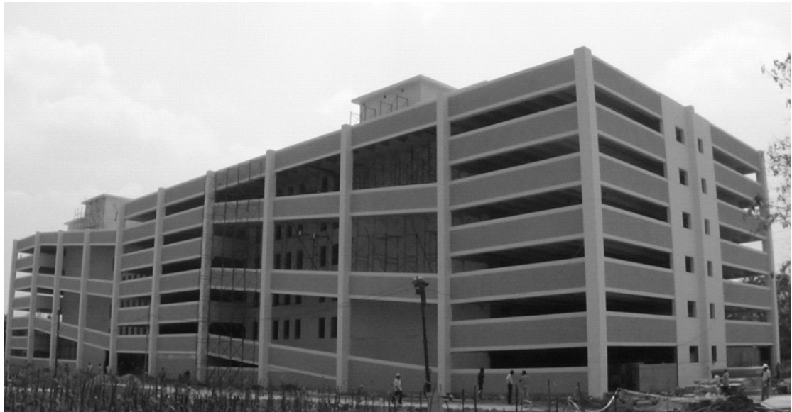
Prefabricated (Precast) MLVP for INFOSYS , MAHINDRA WORLD CITY
