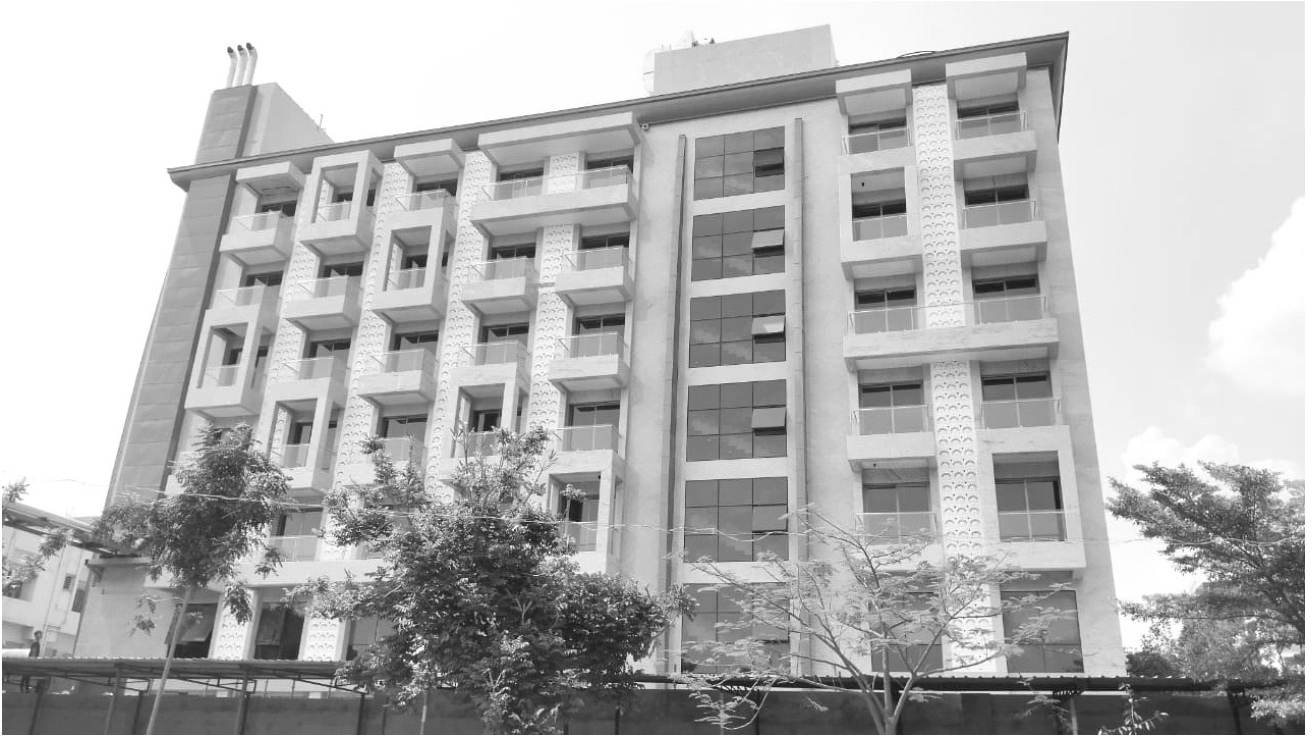
Institutional Building for M/s C.I.S.C.E -Council for the Indian School Certificate Examination (Regional Institute) at Habsiguda, Hyderabad
