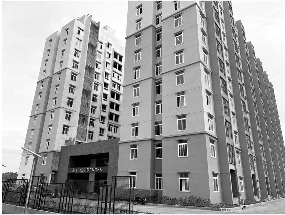
Hostel Building for M/s Dayananda Sagar University at Harohalli, Bengaluru, Karnataka.
