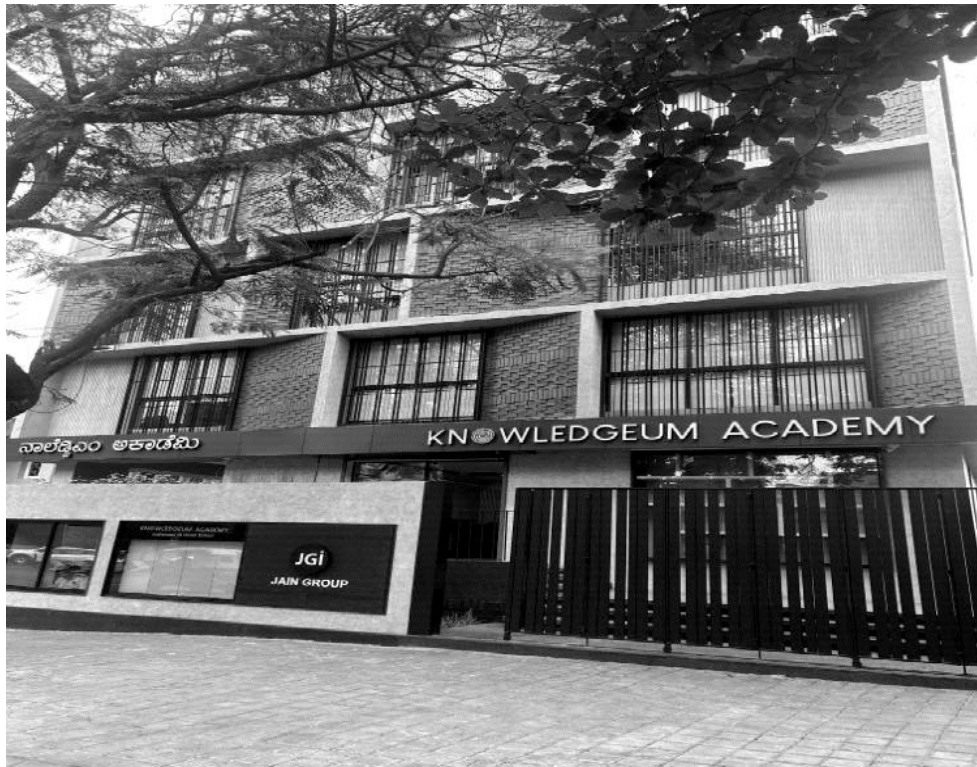
Commercial Building for M/s Sumo Group at Jayanagar , Bengaluru, Karnataka
