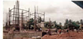
Construction of Manufacturing unit facilities for Lux Flavours at Thirumudivakkam, Chennai
