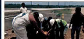
Construction Work for Kitex Apparels Parks Limited at Warangal, Hyderabad
