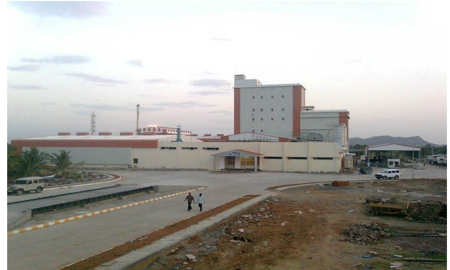
"Factory Building" for Hatsun Agro products Ltd. Kancheepuram
