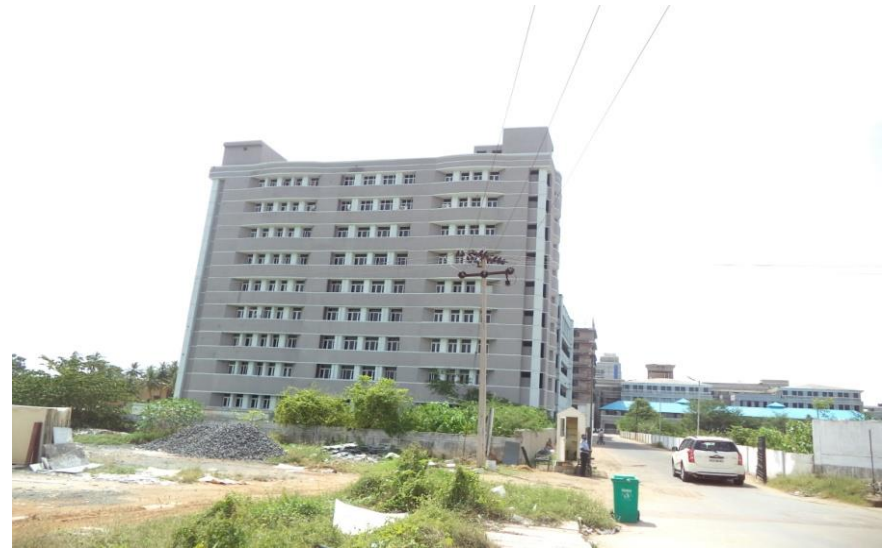
"Institutional Building" for Indira Gandhi Medical College and research Institute, Puducherry
