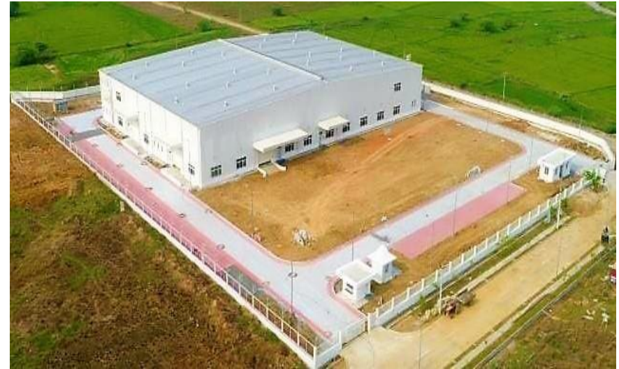
Factory Building for SCL – A Motherson Group Company, Kancheepuram, Tamil Nadu.
