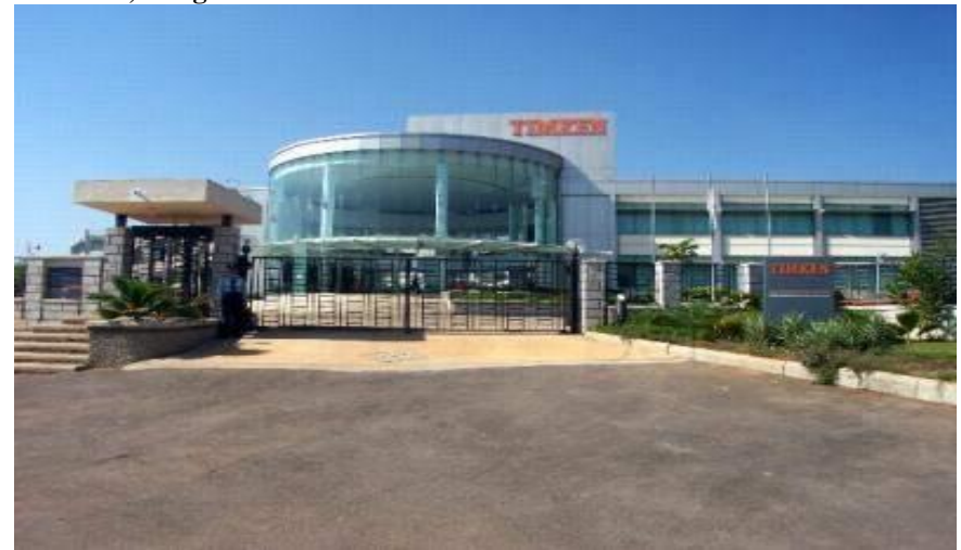
"Factory Building" for Timken Engg & Research (I) Pvt. Ltd, Electronics City, Bangalore
