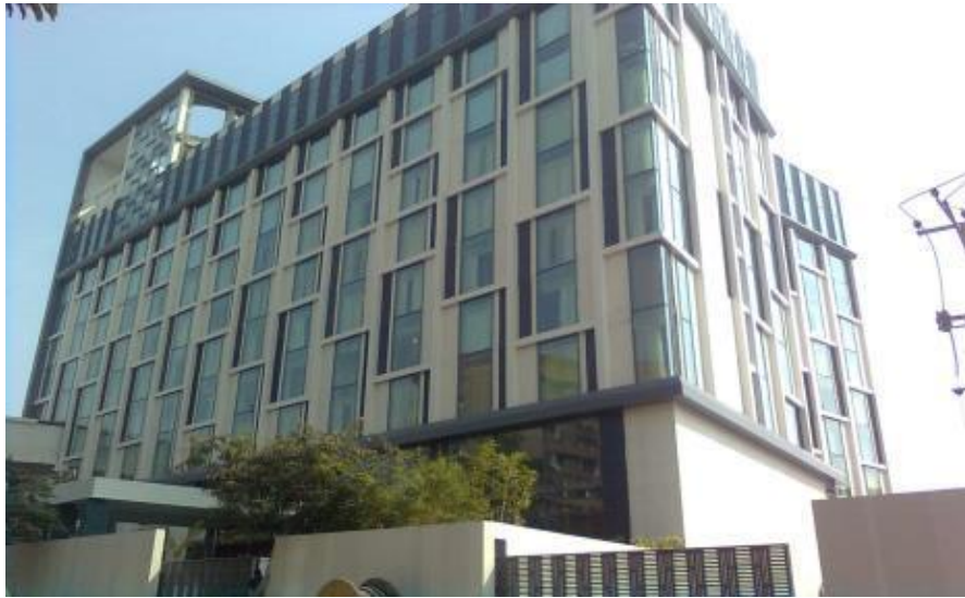
" court yard Building " for Minerva Enterprises Private Limited, Gandhi Nagar, Hyderabad -4 Star 212 Rooms
