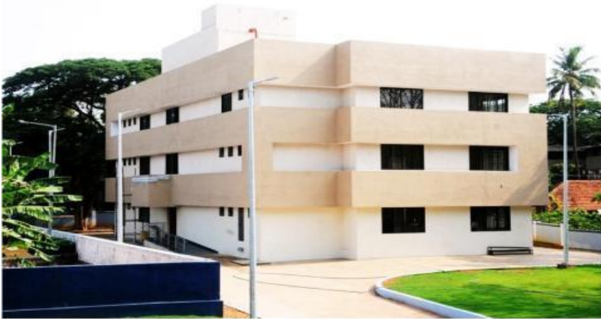
Business Development Park for Export & Testing Centre for New Mangalore Port Trust (NMPT), Panambur, Mangalore
