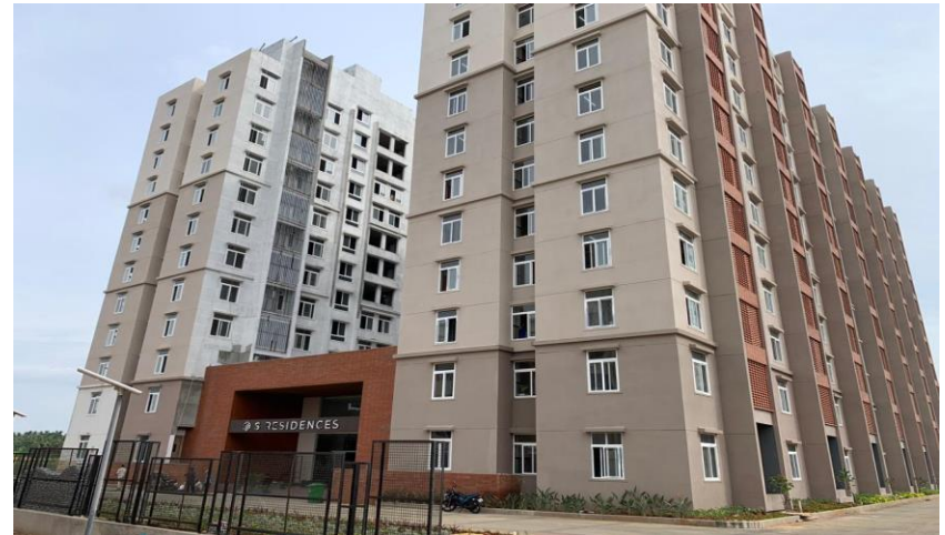
Hostel Building for Dayananda Sagar college of engineering ( Dr. Premachandra Sagar ) , Bangalore, Karnataka.
