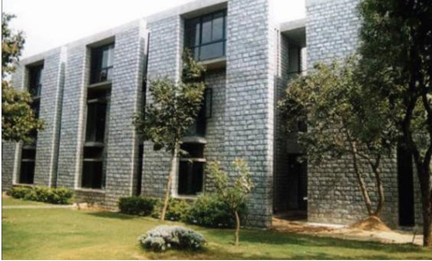
"Institutional Building" for Indian Institute of Management (IIMB), Bannerghatta Road, Bangalore
