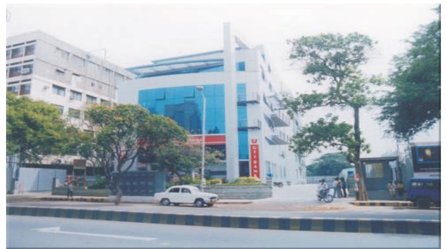
"Commercial Building" for Silver Heights Pvt Ltd, M.G. Road, Bangalore
