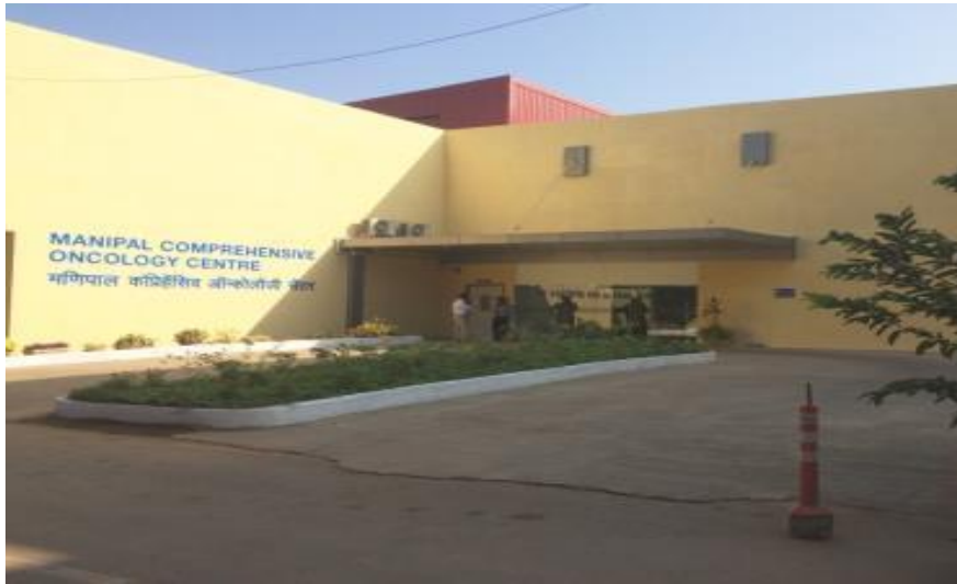
Linac Hospital For Manipal, Panaji, Goa
