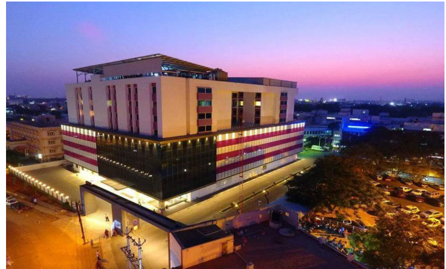
Hospital for Sri Ramakrishna Hospital / SNR Sons Charitable Trust, Avarampalayam, Coimbatore, TN – 400 Beds
