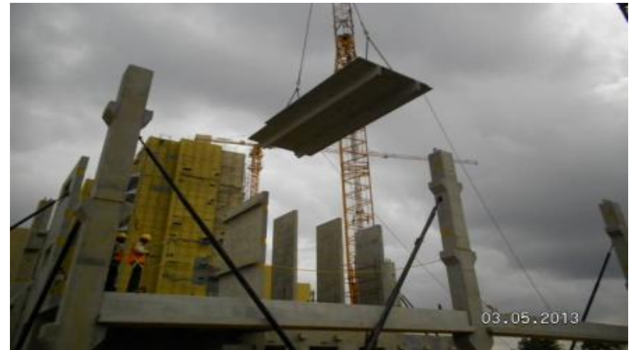
PREFABRICATED DOUBLE TEE SLAB ERECTION
