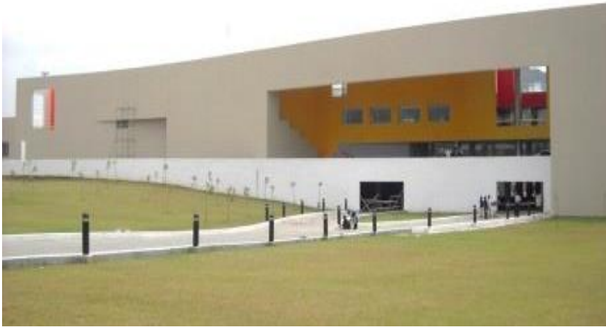
"Product development and Research Centre & other buildings" for (Mahindra Research valley - MRV) Mahindra World City, Chennai
