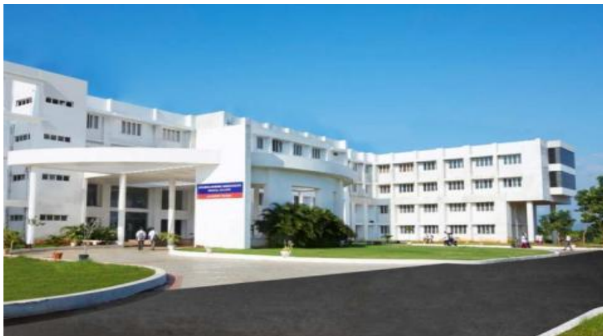
"Dhanalakshmi Srinivasan Medical College" for Dhalakshmi Srinivasan Charitable & Educational Trust, Perambalur – 1000 beds
