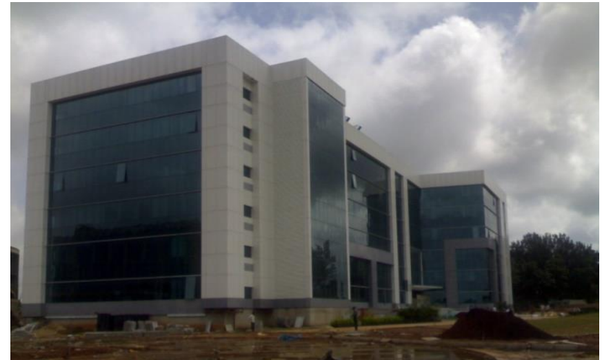
"HCL IT Building" for HCL Technologies Limited, Bommasandra Industrial area, Bangalore
