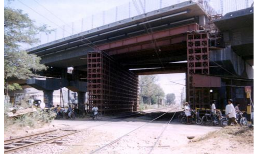
Construction of Rail Over Bridge for Southern Railway, Arakonam , Chennai.
