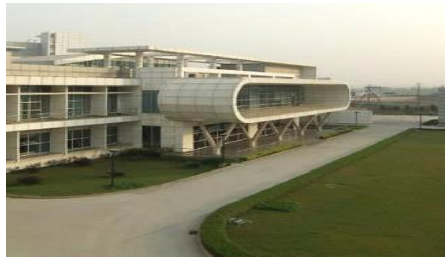
"IT Building" for HCL Technologies Ltd, Noida, UP
