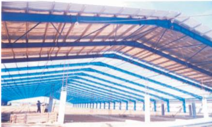
"Factory Building" for Intimate Fashions India Ltd, Guduvanchery, Chennai
