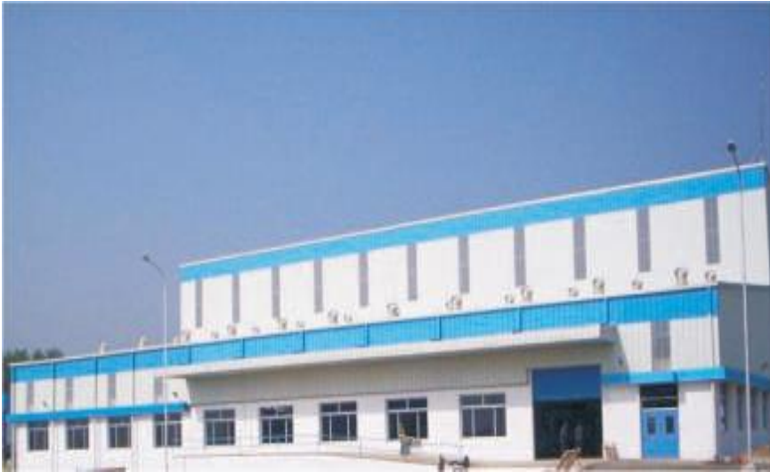
"Construction of buildings and other civil works" for Corborundum Universal Ltd, Uttaranchal
