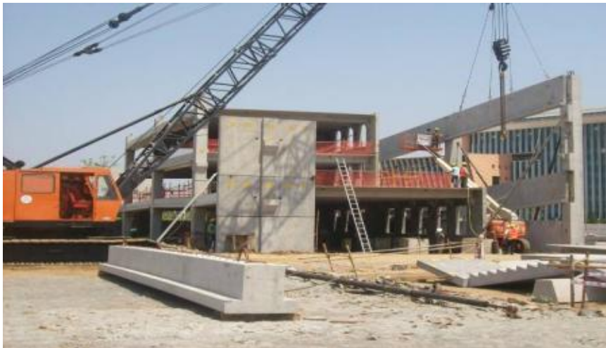
PREFABRICATED SPANDREL ERECTION
