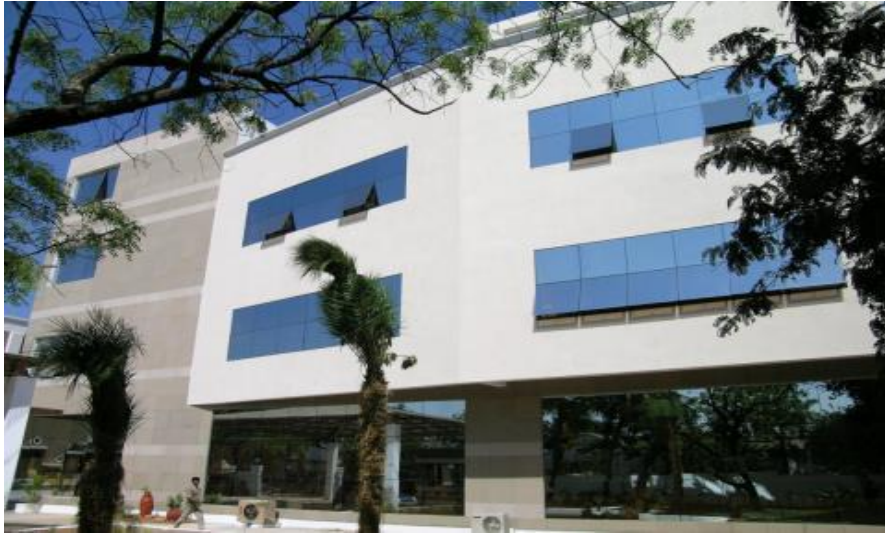
Factory Building for Ambattur Clothing Ltd, Chennai
