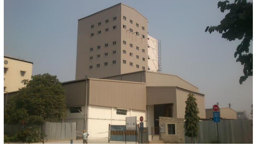
"Civil and structural works at COLT Plant" for Johnson Matthey Chemicals India Pvt Ltd, Kanpur
