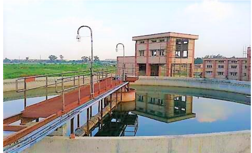
50 MGD Water Treatment Plant for Delhi Jal Board -VA Tech WABAG , Dwarka, New Delhi
