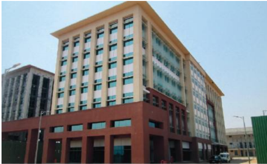
IT Park Building for Infosys, Bhubaneswar, Odisha
