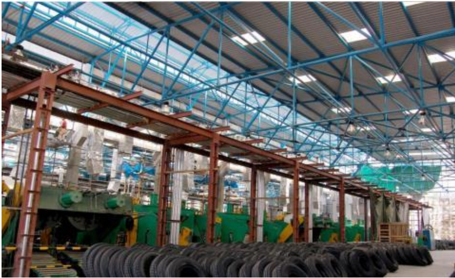
"Expansion work for truck and bus radial tyre plant" for J K Tyres and Industries Ltd, Hebbal Industrial Area, Mysore
