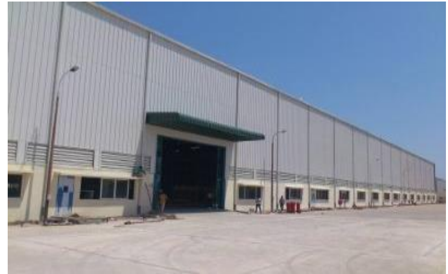
"Factory Building" for Schwing Stetter India Pvt Ltd, Irungattukottai, Chennai
