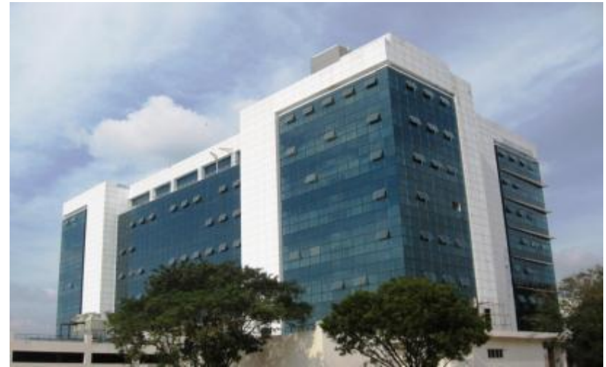
"Internet Data Centre Complex" for TATA Communications Pvt Ltd, Ambattur, Chennai
