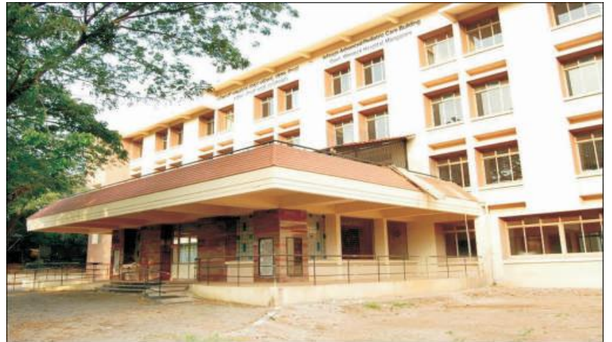
"Wenlock Hospital" for Infosys Foundation, Hampankatta, Mangalore
