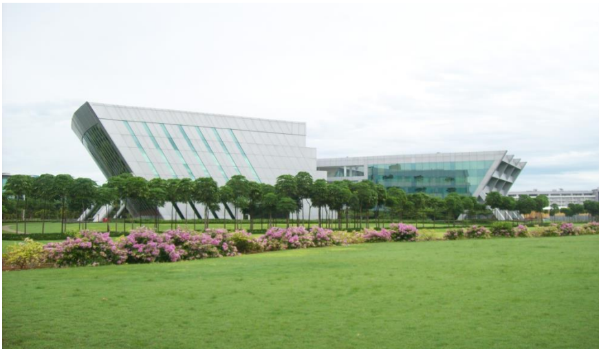
"Software Development Block (SDB-3)" for Infosys Technologies Ltd, Mahindra World City, Chenglepet, Near Chennai
