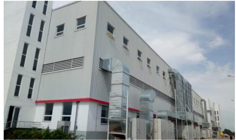
SMR Factory Building for Motherson Group ,Walajabad, Kancheepuram
