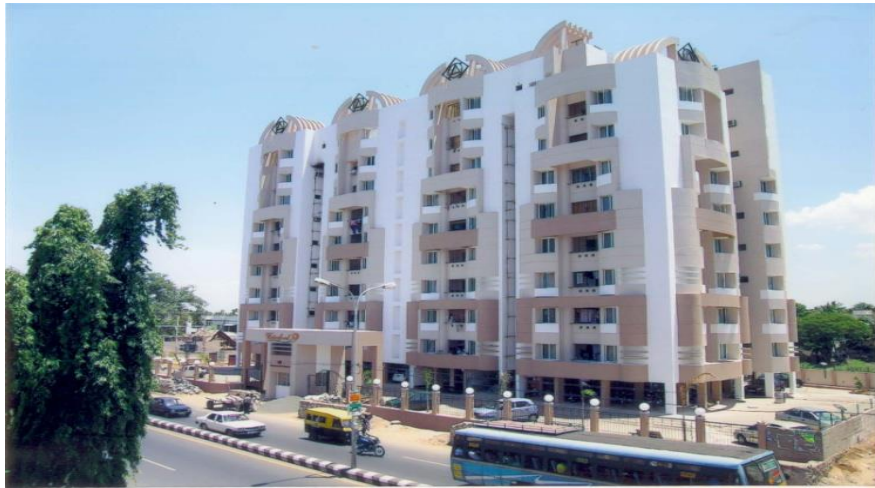
"SAS Water Ford - Residential Building" for SAS hotels & enterprises, Thiruvanmiyur, Chennai
