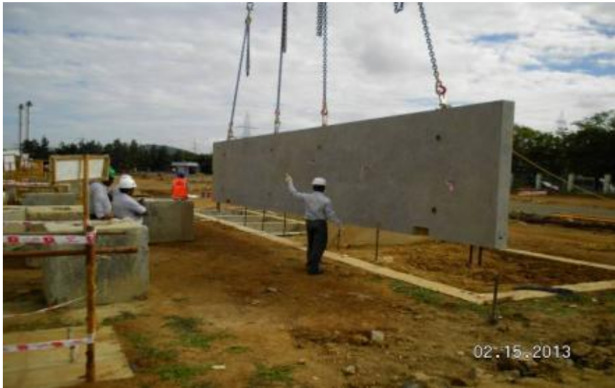
PREFABRICATED LIFT WALL PANEL ERECTION
