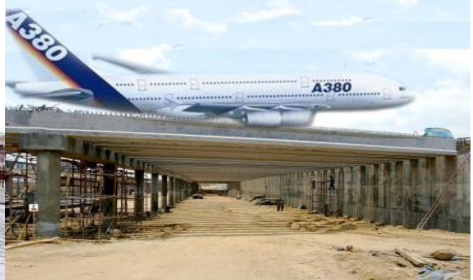
RCC/Pre-stressed concrete bridge for aircraft movement across the adyar river for Airports Authority of India (AAI), Adayar, Chennai, Tamil Nadu
