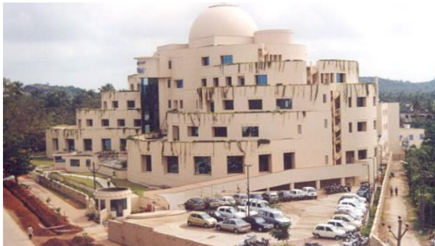
"Software Development Block (SDB)" for Infosys Technologies Ltd, Kottara, Mangalore, Karnataka
