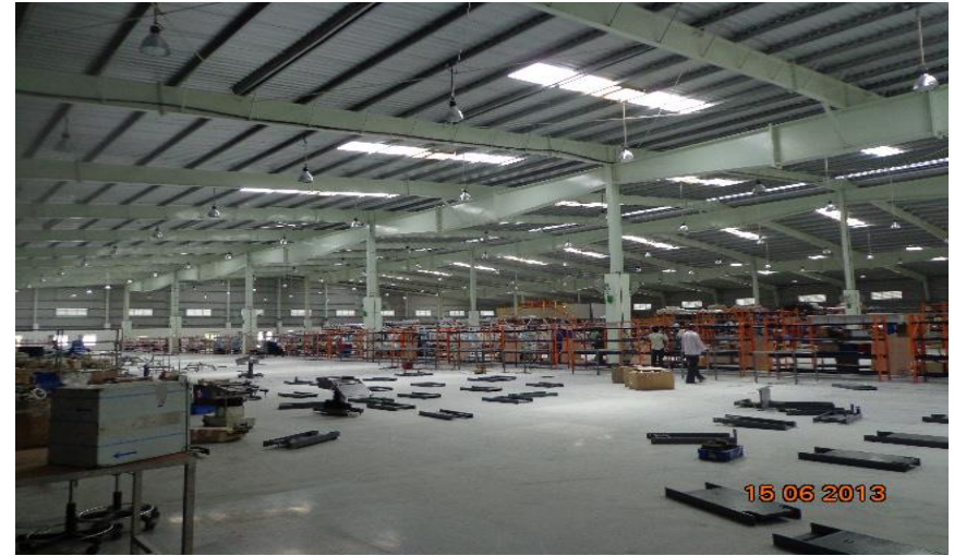
"Factory Building" for Confident Dental Equipment, Bidadi Industrial Area, Bangalore
