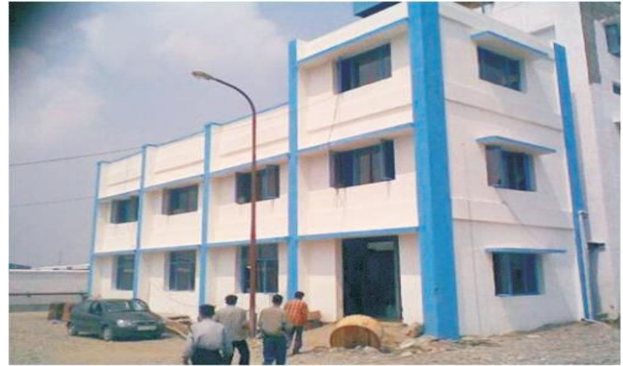
"Factory Building" for SRF Polymers Ltd, Rudrapur, Uttarakhand
