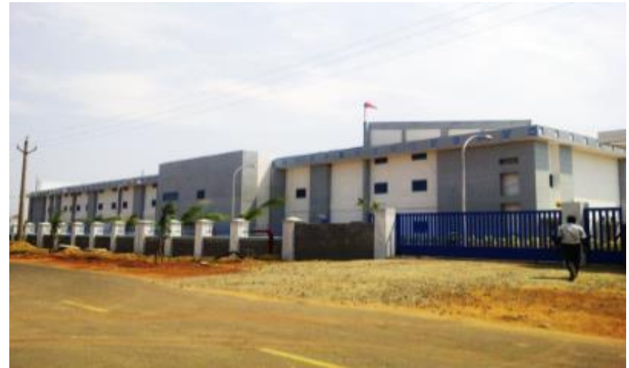
"OSD Formulation plant" for Til Exports Pvt Ltd. (Tablets India) Sricity, SEZ, TADA.
