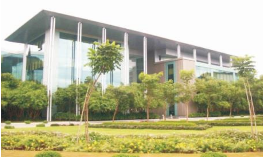
"Software Development Block (SDB-1)" for Infosys Technologies Ltd, Mahindra World City, Chengalpet, Near Chennai
