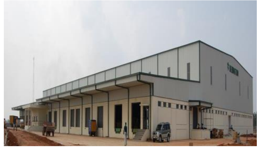
Ware House Utility & Ancillary Building for Redington (India) Limited, Gummidipoondi, Chennai
