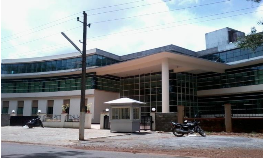
Administration building for T.A.Pai Management institute(School of management) For manipal university, Manipal, Karnataka
