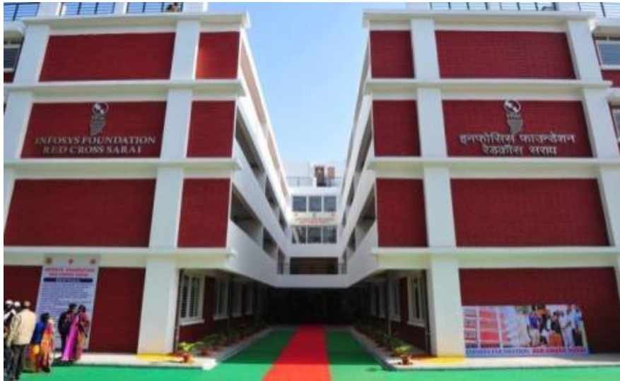
Infosys Redcross Sarai P.G.I.M.E.R- Campus Dharmashala Building, Chandigarh ,Punjab
