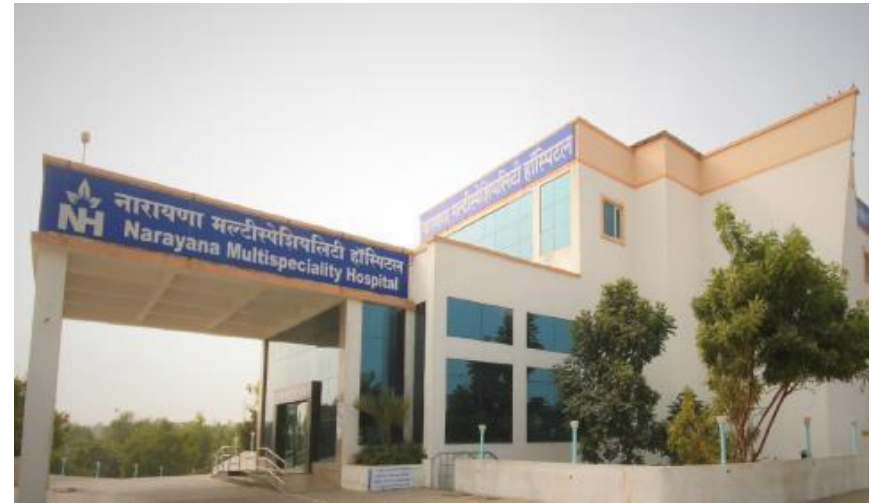
"Multispeciality Hospital" for Narayana Hospital private Ltd., Jaipur – 290 Beds
