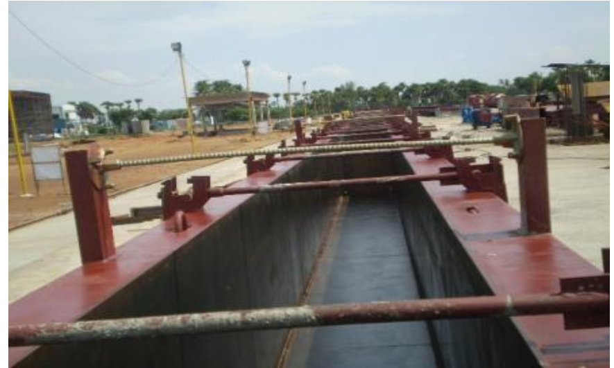
PRODUCTION LINE COLUMN MOULD
