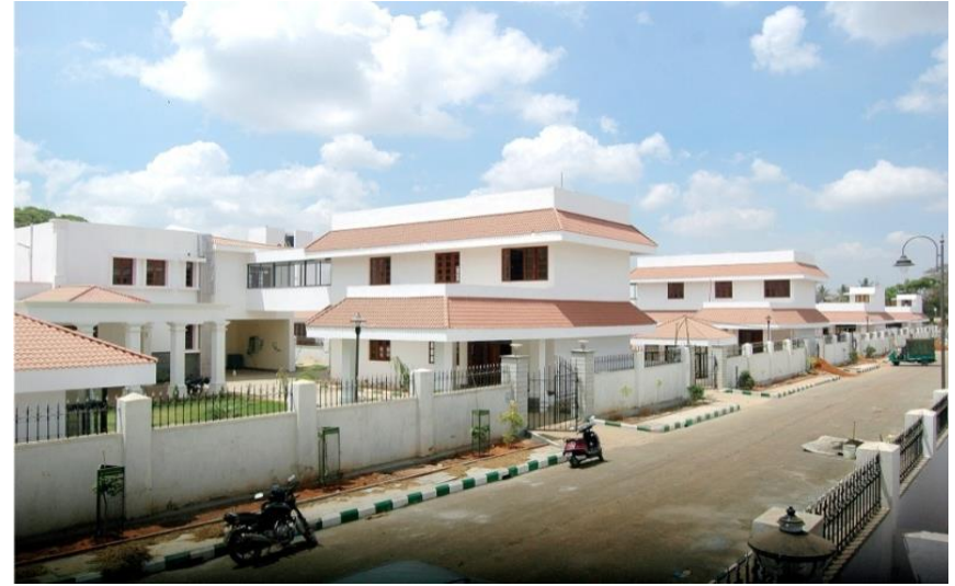
"Ministers Quarters - Residential Building" for Govt. of Karnataka, Karnataka
