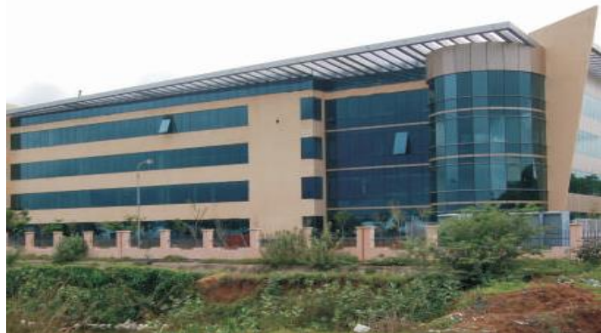
"IT Building" for Mastek Ltd, Mahindra World City, Chenglepet, Near Chennai
