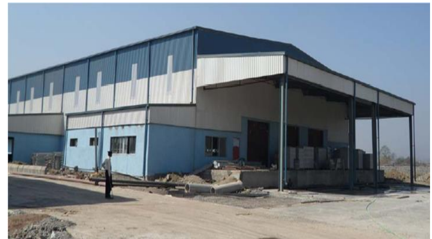
"Paint Manufacturing Plant" for Nippon Paints Pvt Ltd., Talaja, Pune
