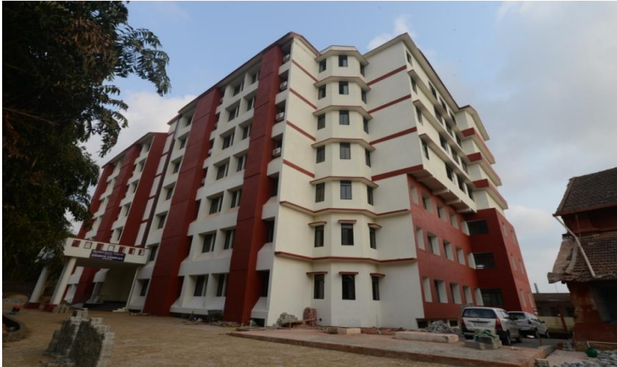
"District Court Building " for Karnataka Public works Department, Court Hill, Mangalore
