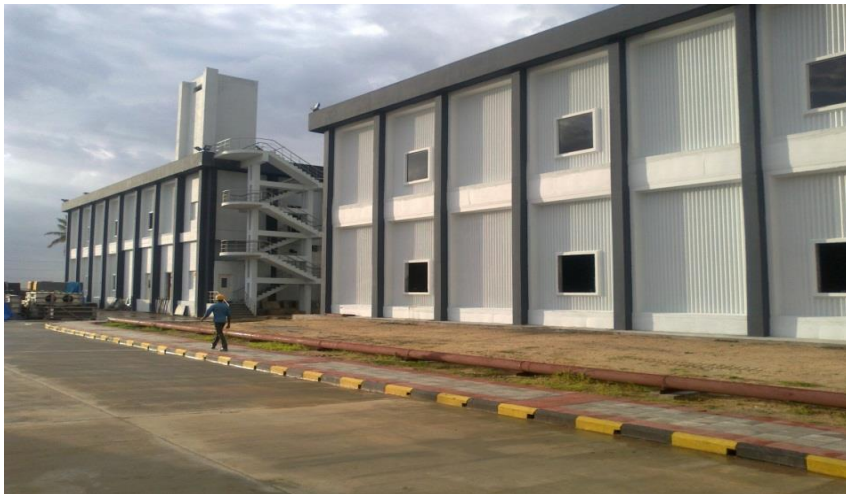
"Pharma plant with Precast Wall Panels" for Shantha Bio technics Pvt Ltd, Medchal, Hyderabad
