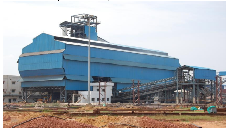
"Mini Blast furance plant" for SBQ Steel Ltd, Nellore, Andhrapadesh
