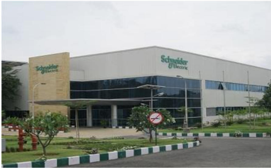
Manufacturing Facility for Schneider for Essae-Teraoka Pvt Limited, Attibela Industrial Area, Karnataka
