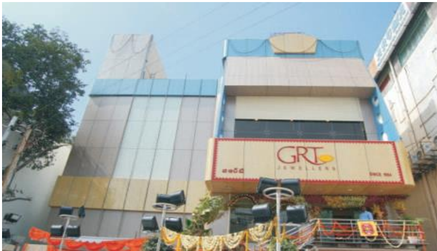
"Commercial Building" for G.R.Thangamaligai Pvt. Ltd, Somajiguda, Hyderabad
