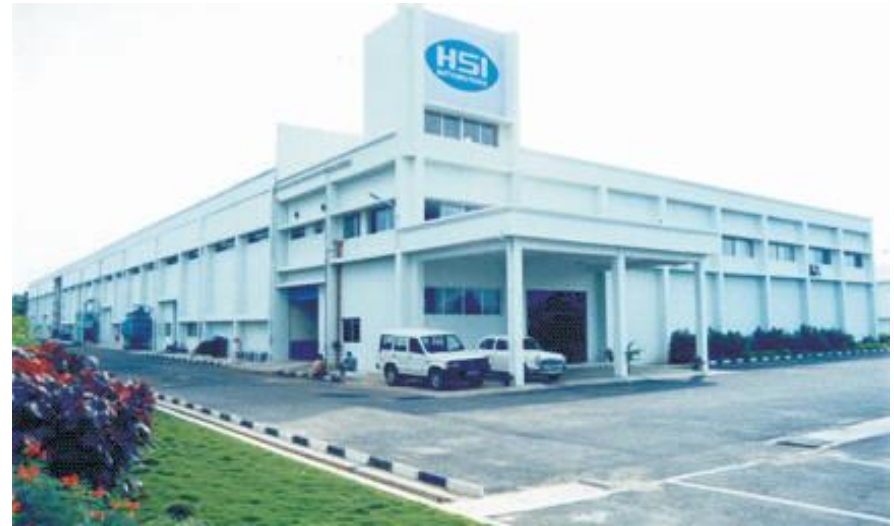
"Factory Building" for HSI Automotive India Ltd, Chevillimedu, Chennai
