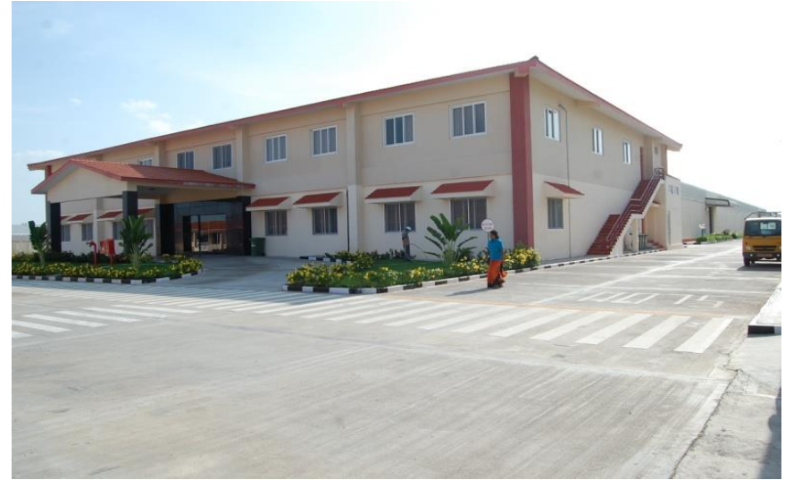
"LU2 / LU3 Building works" Cheyyar SEZ Developers Private Limited, Cheyyar, Tiruvannamalai District
