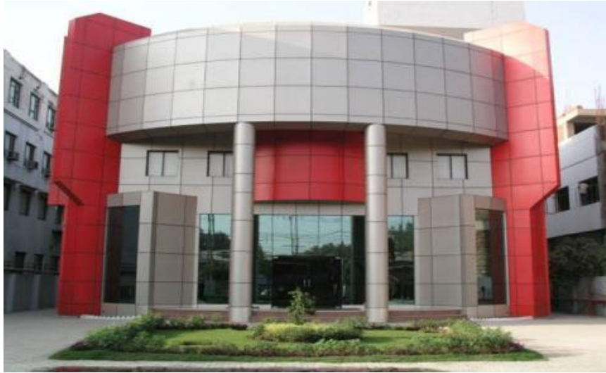
"Show Room and Service centre" for MRF Ltd, New Delhi
