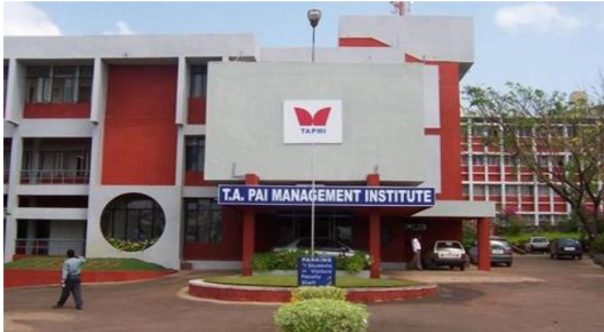
Construction of TAMPI Management Block for T A Pai Management Institute, Manipal, Karnataka
