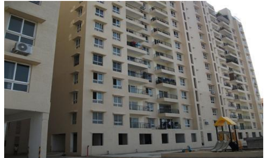
Plama Heights Apartments for "Plama Heights" Residential and Commercial Development, Kosaba hobli, Bangalore
