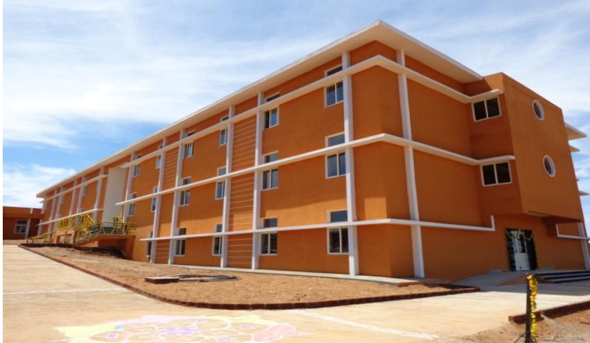
"Infosys Isha Vidhya School Building" for Infosys Technologies Limited, Dharmapuri
