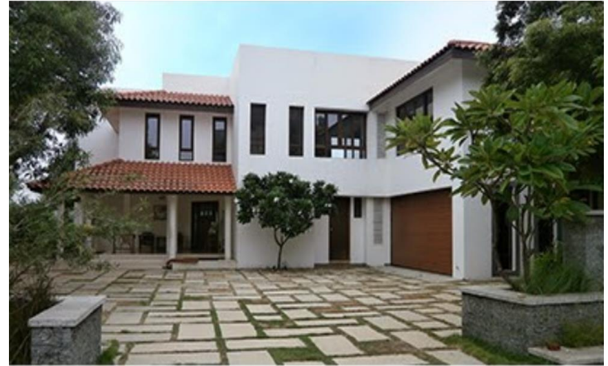
Buckingham Garden - Phase 2 for Raj water scape Properties Pvt Ltd ECR Road, Kanathur, Chennai
