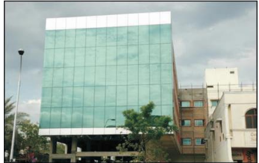
"Office Building" for Silpa Electricals, Choolaimedu, Chennai
