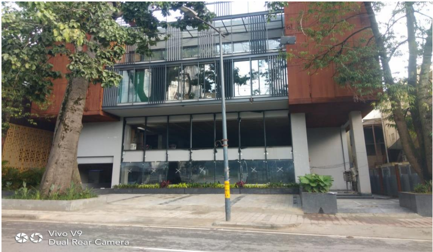
Office Space Building for Shruthi Builders, Cunningham Road, Bangalore
