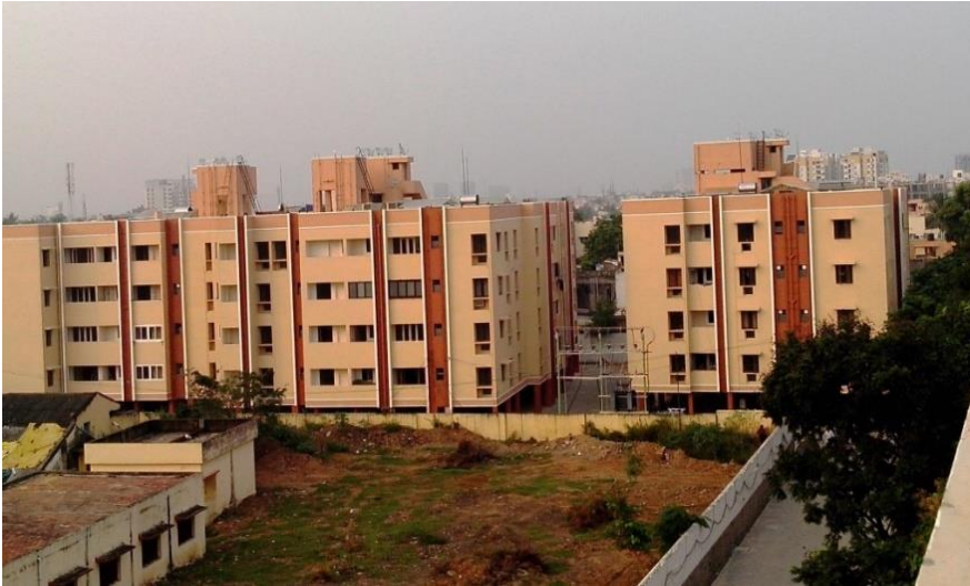
"Residential Building Yuga Kalpataru" for Yuga Homes(CCCL), Chennai
