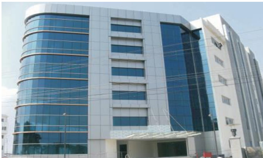
"IT Building" for Daya Cyber Park Ltd, Near Mattuthavani Bus Stand, Madurai
