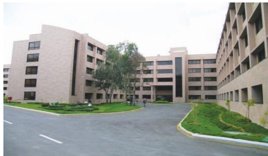
"Hostel Building" for Infosys Technologies Ltd, Hebbal Industrial area, Mysore
