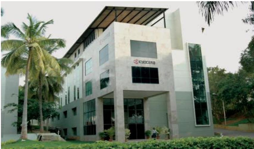
"Kyocera Technologies - Commercial Building" for Tangling Developers Ltd, Global Village, Mysore Road, Bangalore
