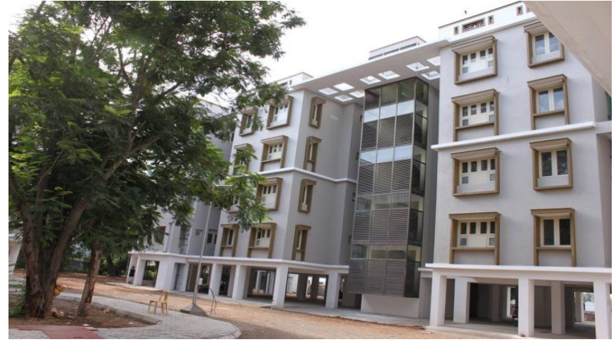
"C & D type Quarters in Sunset Avenue at CMC" for Christian medical college, CMC, Bagayam Campus, Chennai
