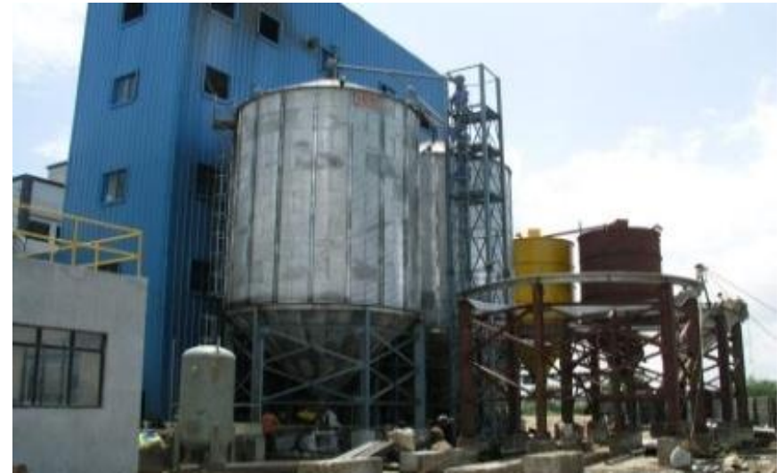
"Brewery modernisation" for Skol Breweries Ltd, Hyderabad
