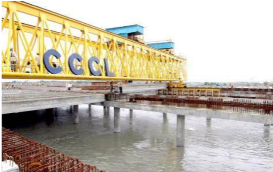
RCC/Pre-stressed concrete bridge for aircraft movement across the adyar river for Airports Authority of India (AAI), Adayar, Chennai, Tamil Nadu
