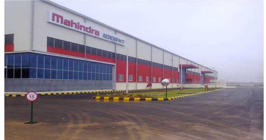
"Manufacturing Plant" for Mahindra Aerostructures Pvt Ltd, Industrial Area Narasapura, Kolar District, Karnataka
