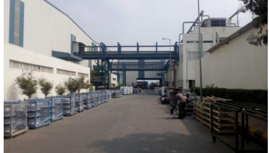
Factory Building (Phase 2) for Steel Strips Wheels Ltd, Oragadam, Chennai
