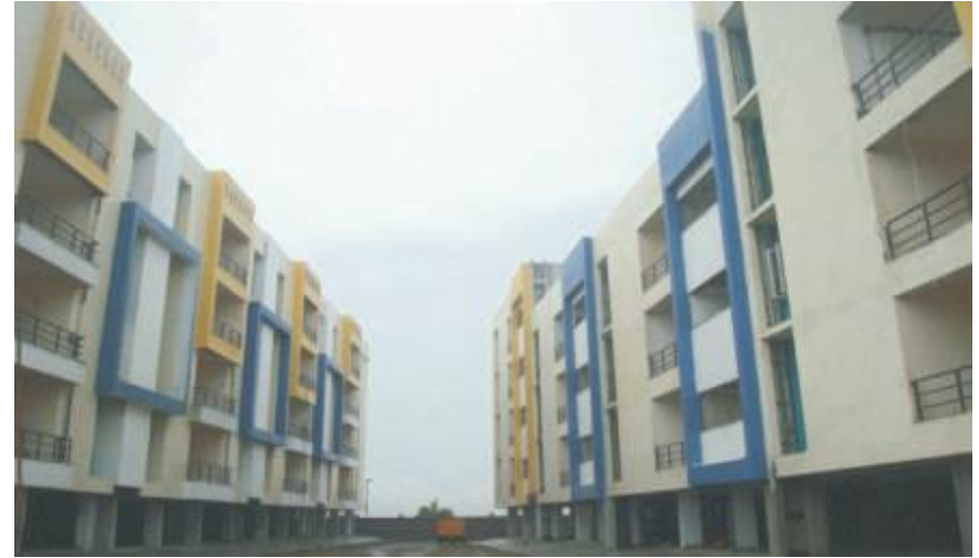
"Shem Park - Green Homes Gold Rated Green Building" for Yuga Homes Ltd, Chemmenchery, Chennai
