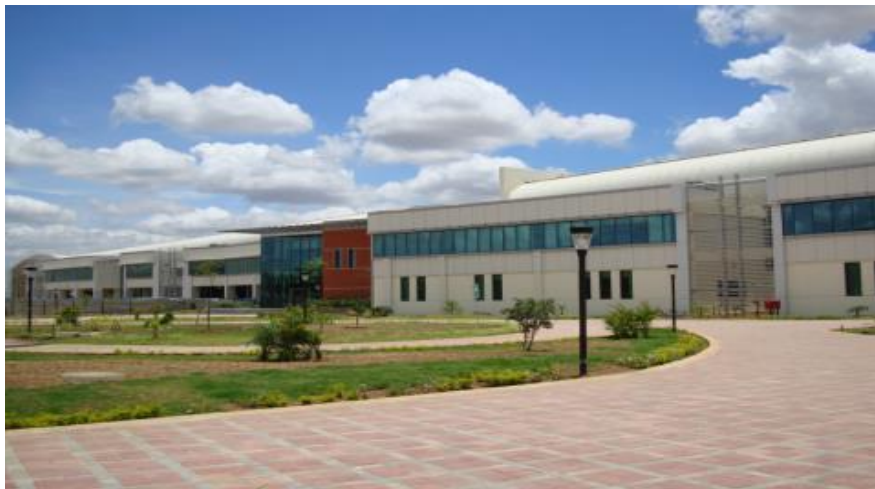
"Factory Building" for ITC Limited, Pune
