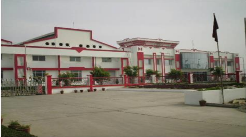
"Dry Cell Manufacturing Plant" for Eveready Industries India Ltd, Haridwar, Uttarakhand
