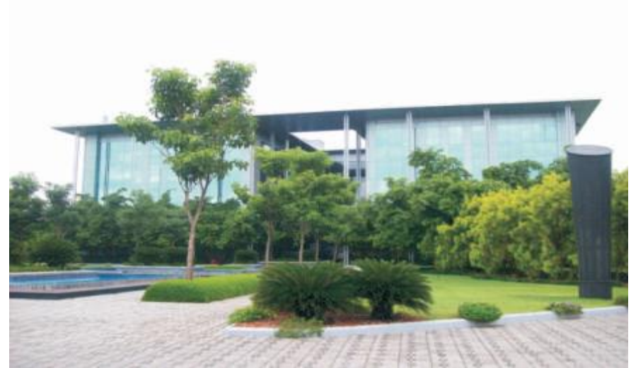
"Software Development Block (SDB-2)" for Infosys Technologies Ltd, Mahindra World City, Chengalpet, Near Chennai
