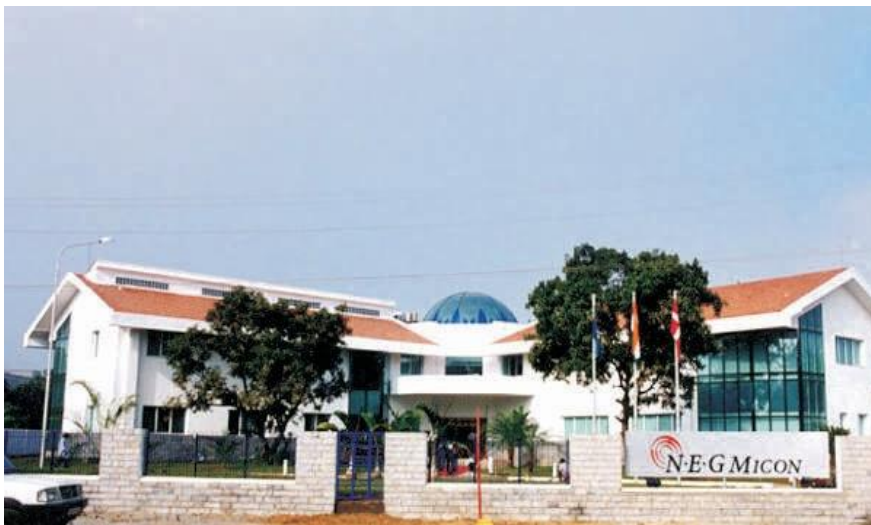
"Gold Rated Green Building" for NEG Micon (Now "Vestas" ), Sholinganallur, Chennai
