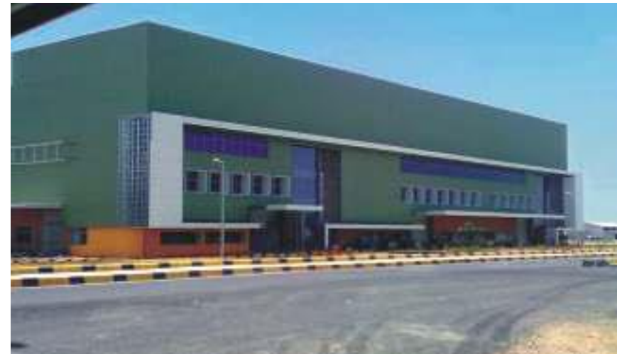
"Land development work" for Mahindra Automotive Ltd, MIDC Chakan, Pune
