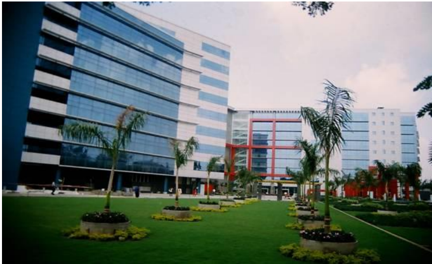
"Olympia Technology Park" for Khivraj Tech Park Pvt Ltd, Guindy, Chennai -LEED Gold Rated Green Building (USGBC)
