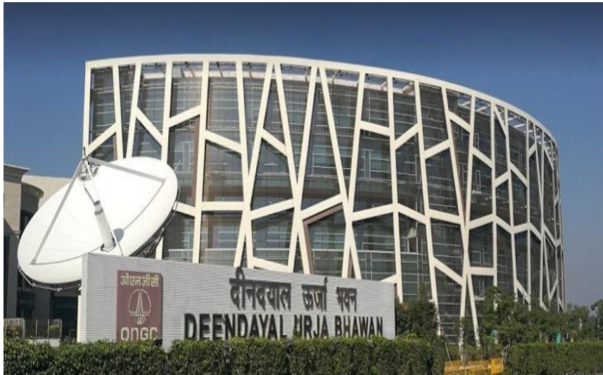
"Rajiv Gandhi Urja Bhawan" for ONGC ( Energy Centre and Corporate Office), Delhi
