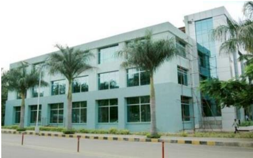
"IT Building" for Texas Instruments India Pvt Ltd, Global Village, Mysore Road, Bangalore
