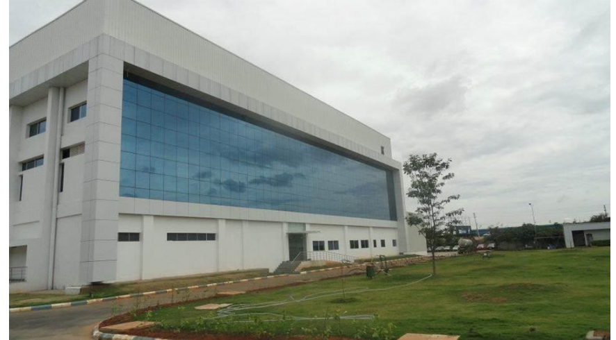
"Pharmaceutical Building" for Kemwell Pvt Ltd, Tumkur Road, Bangalore
