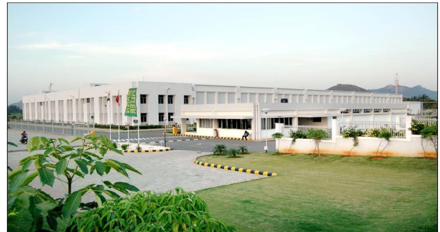
"Manufacturing Plant" for Mann & Hummel Filter Pvt. Ltd, Antharasanahalli Industrial Area, Tumkur, Bangalore, Karnataka
