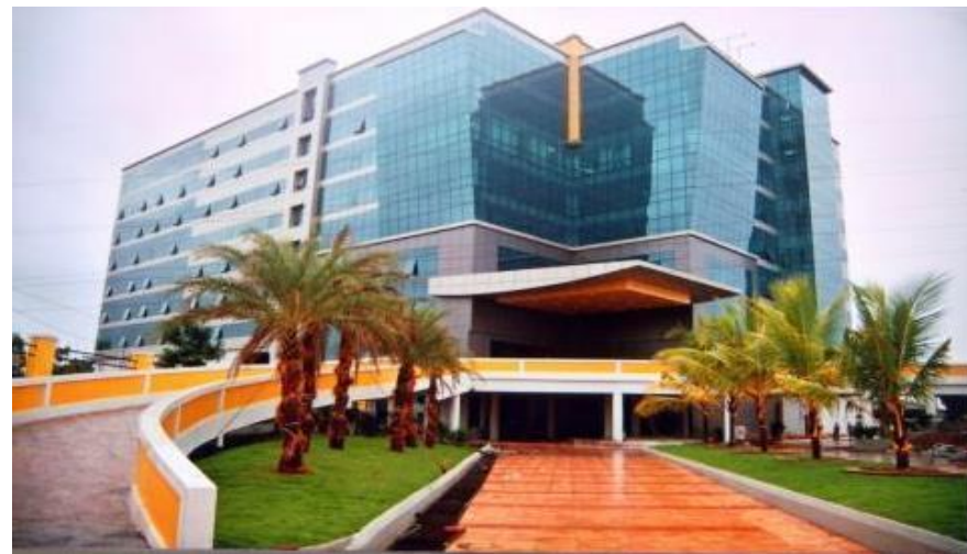
"Technopolis - IT Building" for Muthoot Hotels & Tourism Venture Pvt Ltd, Kakkanad, Kochi
