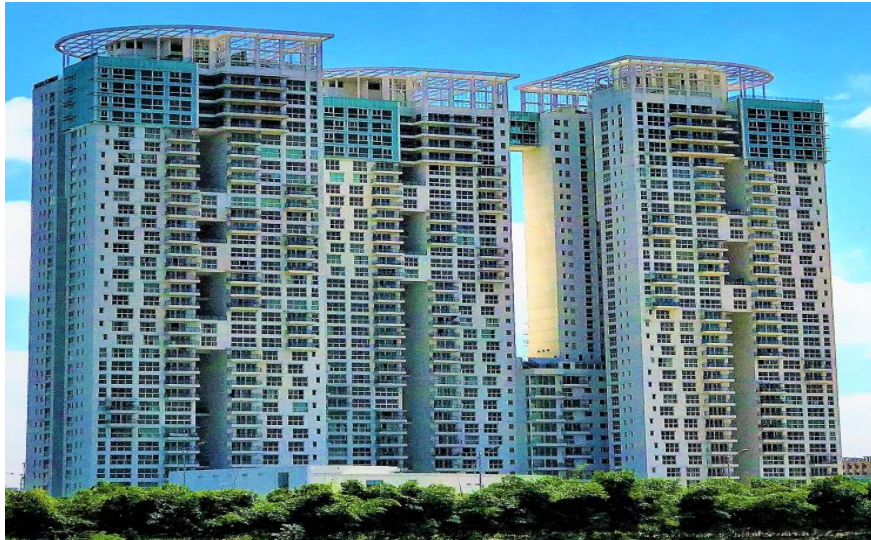
Zenith Towers for Karle Homes Pvt Ltd, Bangalore, Karnataka
