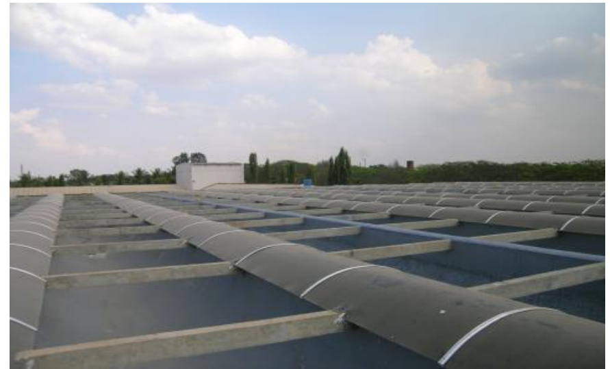
Factory Building for Rittal India Pvt Ltd, Doddaballapur, Bangalore
