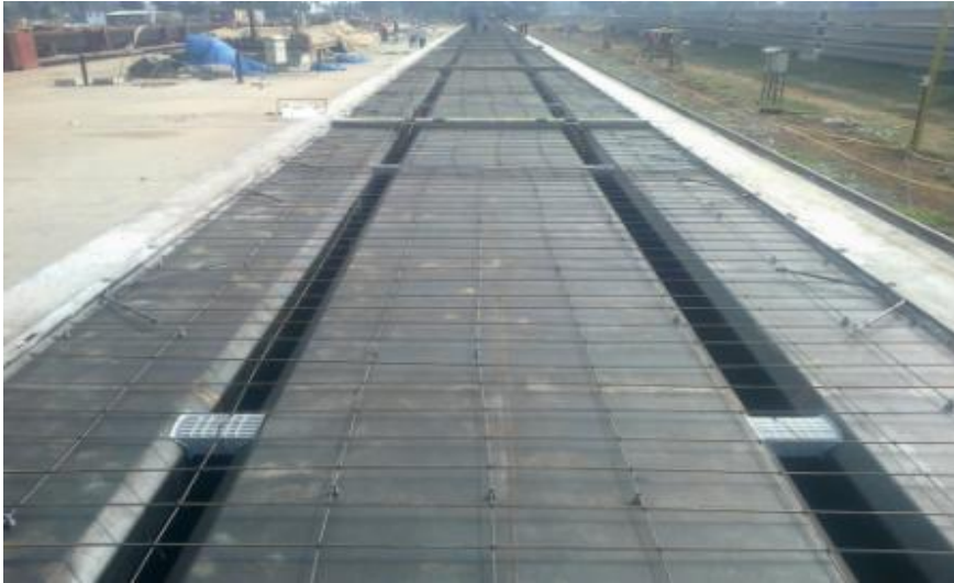
PRODUCTION LINE DOUBLE TEE MOULD
