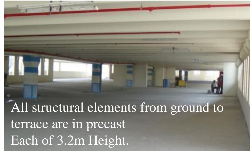
Precast Multi Level Two Wheeler Parking – MLVP for Infosys, Mahindra City SEZ Campus, Chennai 3683 Nos – 2 Wheeler Parking's
