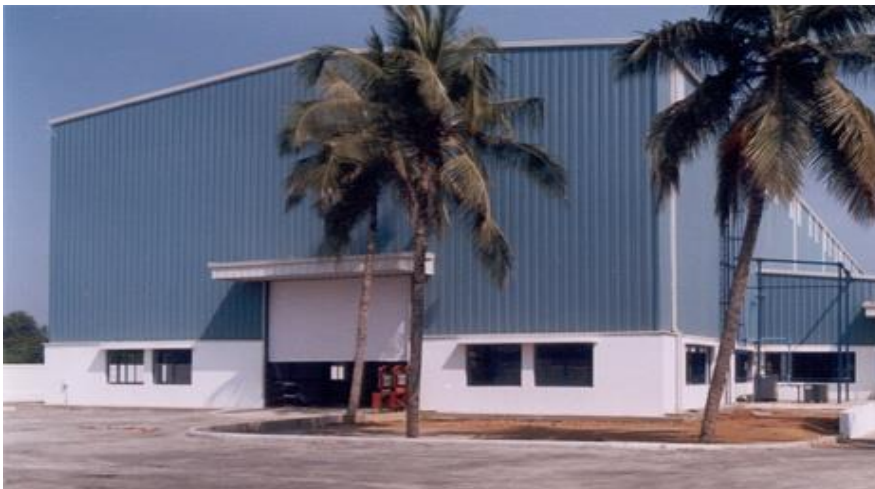
Warehouse Building for Neg Micon (I) Pvt Ltd (Vestas Wind Technologies India Pvt Ltd), Thiruvandarkoin, Puducherry
