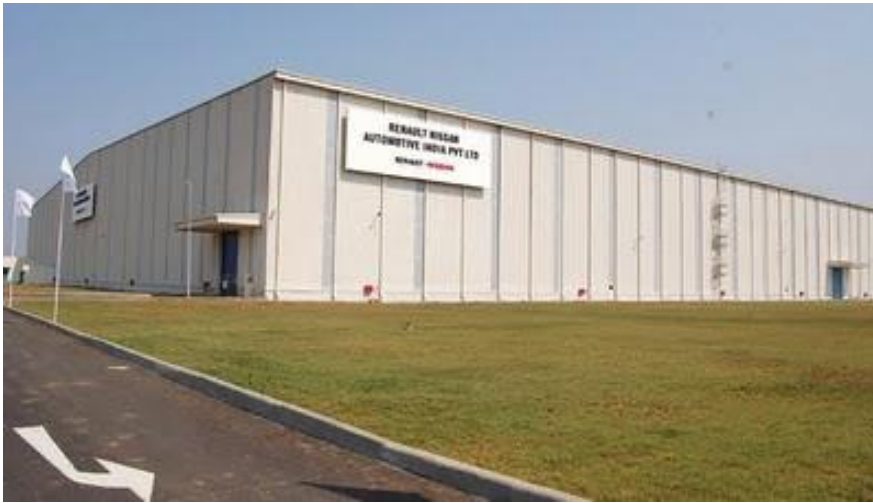
"Renault Nissan Unit with Boundry Fencing" for Renault Nissan Motors Co. Ltd, Oragadam, Chennai
