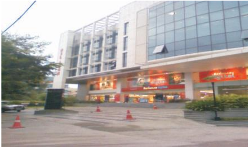
"Commercial Building" for Nuziveedu Seeds Ltd, Banjara Hills, Hyderabad
