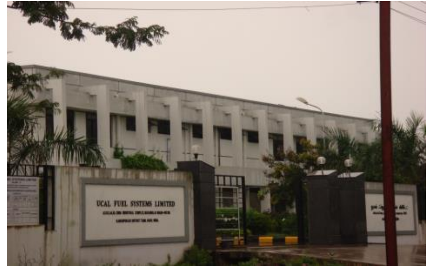
Factory Building for UCAL Fuel system Ltd, Mahindra SEZ, Chengalpet, TN
