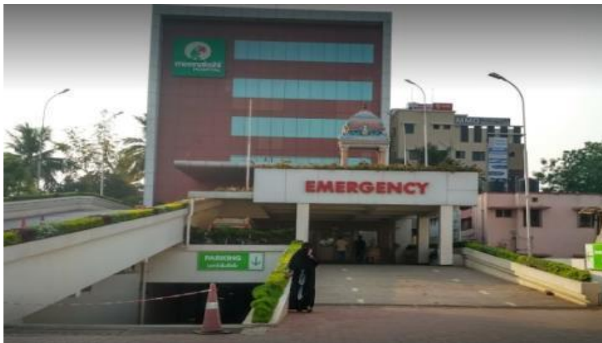
Madurai Meenakshi Hospital, Thanjavur, TamilNadu – 250 Beds
