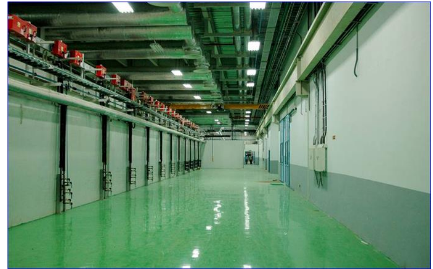
"Industrial Manufacture Building on (Phase 2)" for Foxconn India Pvt. Ltd, Irungattukottai, Chennai
