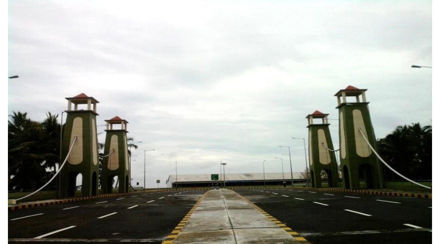
Trivandrum Airport Ramp Work connecting bridge over chackal canal and car park, Kerala
