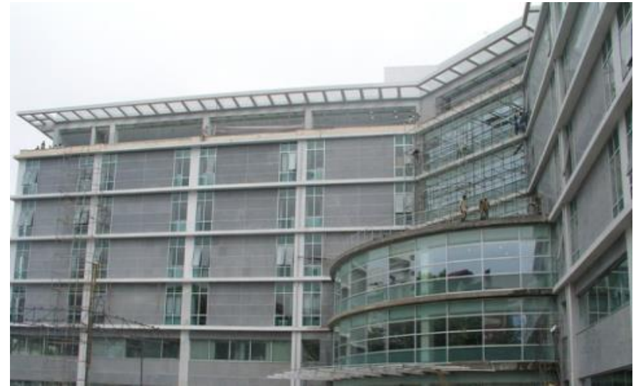
"IT Building" for Motor Industries Co Ltd (MICO), Koramangala, Bangalore
