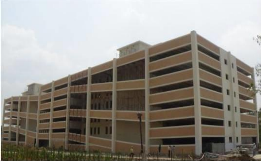
Precast Multi Level Two Wheeler Parking – MLVP for Infosys, Mahindra City SEZ Campus, Chennai 3683 Nos – 2 Wheeler Parking's
