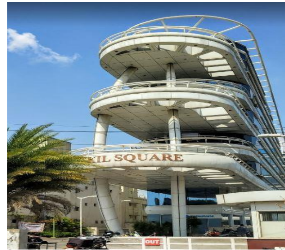
Vakil Square ( Office ) for Vakil Housing Development Corporation, Bannerghatta Road , Bangalore
