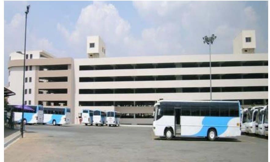
"Multilevel Car Park (MLCP)" for Infosys Technologies Ltd, Electronics City, Bangalore
