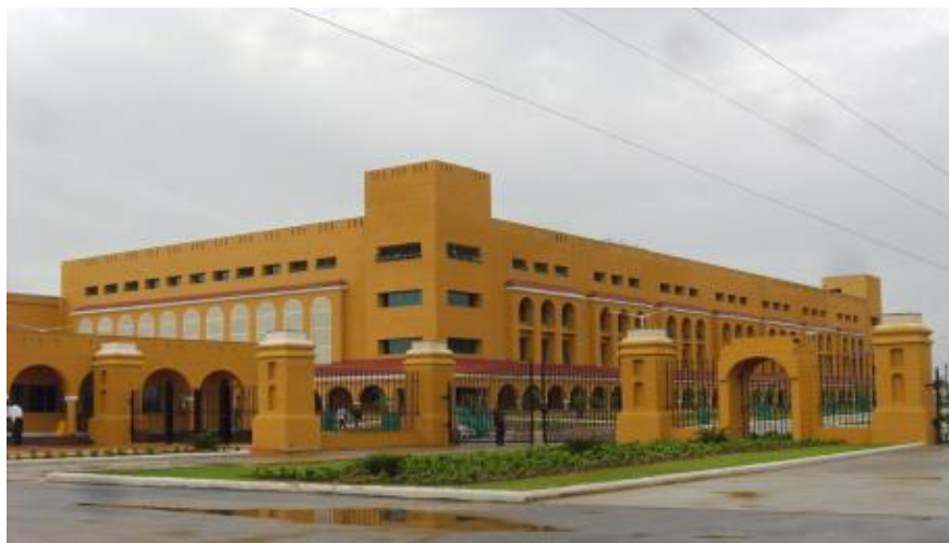
"Administration - Library" for Manipal International University Jaipur
