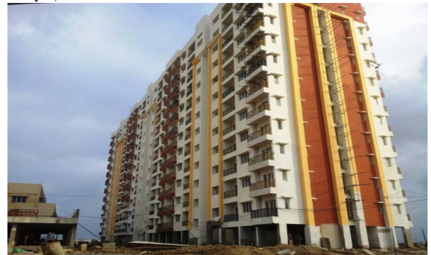
"Alta Vida Residential Building" Yuga Homes(CCCL),OMR, Thaiyur, Chennai
