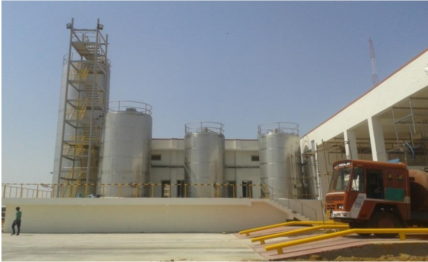
"Dairy Plant" for Hatsun Agro Product Ltd, Aayaneri Village, Tirunelveli
