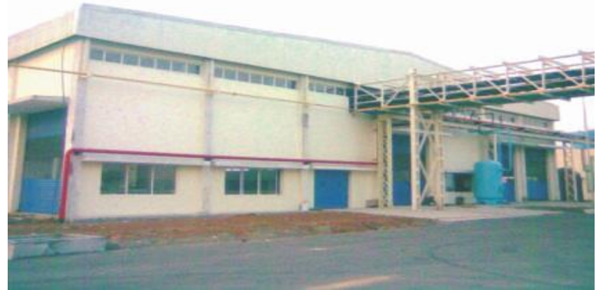
"Factory Building" for Steel Strips Wheels Ltd, Sriperumpudur, Chennai
