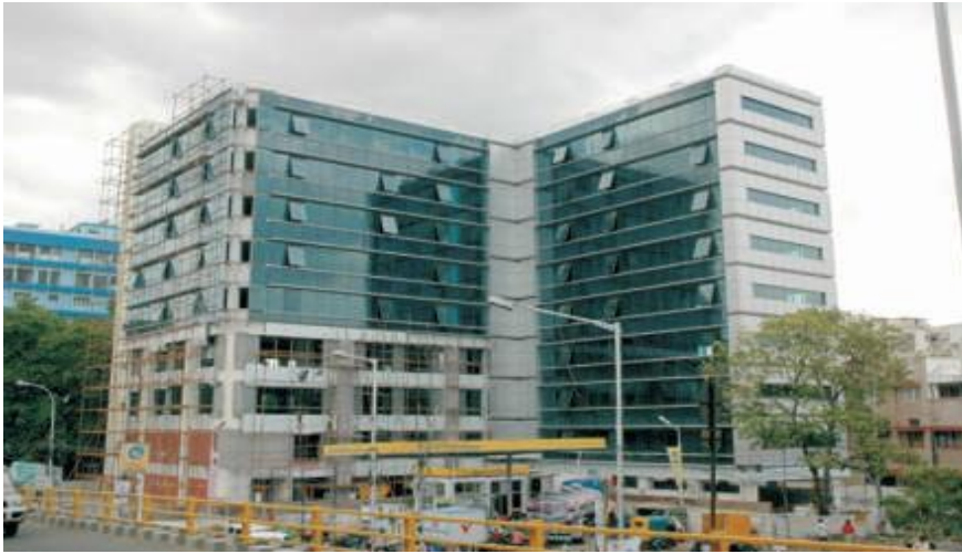
"Samson Tech Park - Commercial Building" for Samson Foundation, Egmore, Chennai
