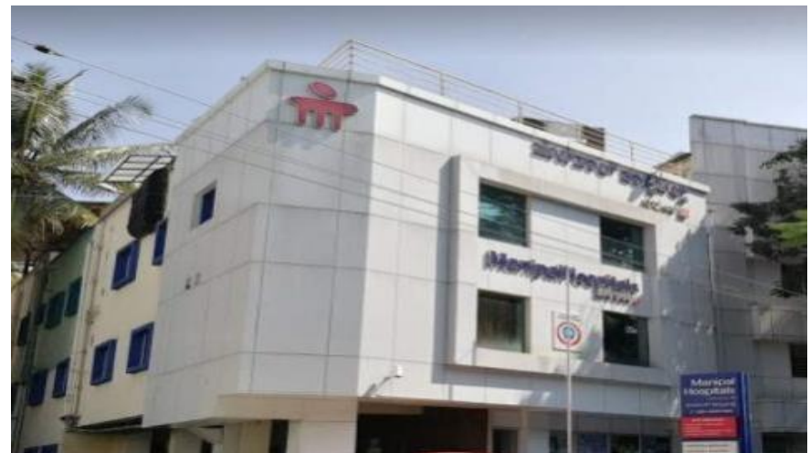
Manipal North Side Hospital For MEMG International India Pvt. Ltd, Malleswaram, Bangalore - 85 Beds
