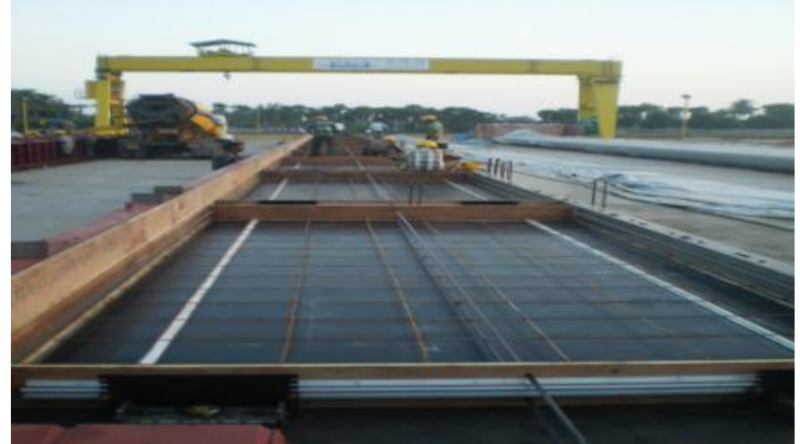
PRODUCTION LINE WALL
