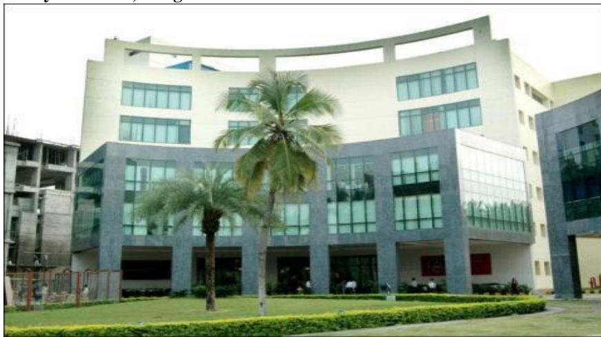
"Mind Tree IT Park (Phase - 2)" for Tanglin Developers Ltd, Global Village, Mysore Road, Bangalore
