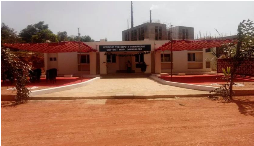
"CISF Township –Office Building" Mangalore Refinery and petro chemical Ltd., Mangalore
