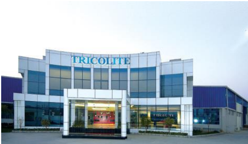
"Tricolite - Electrical Pannels" for Tricolite Electrical Industries Pvt. Ltd, Gurgaon, Haryana
