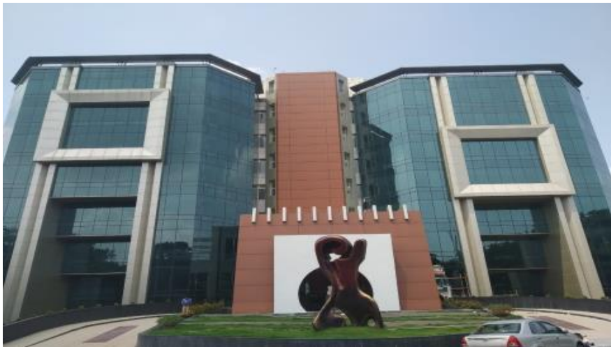
Construction of Multi Level Car Parking Building for Oil and Natural Gas Corporation Ltd, Tel Bhawan, Dehradun
