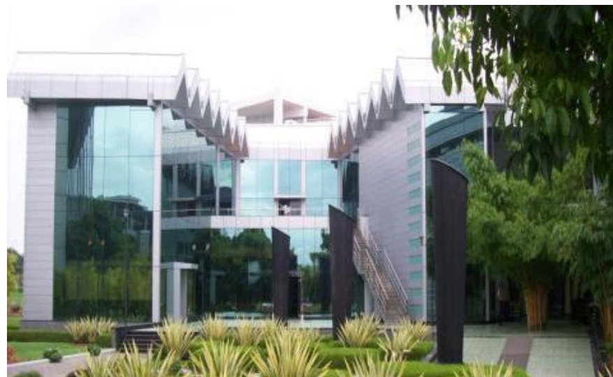
"Foodcourt for SDB-1" for Infosys Technologies Ltd, Mahindra World City, Chenglepet, Near Chennai
