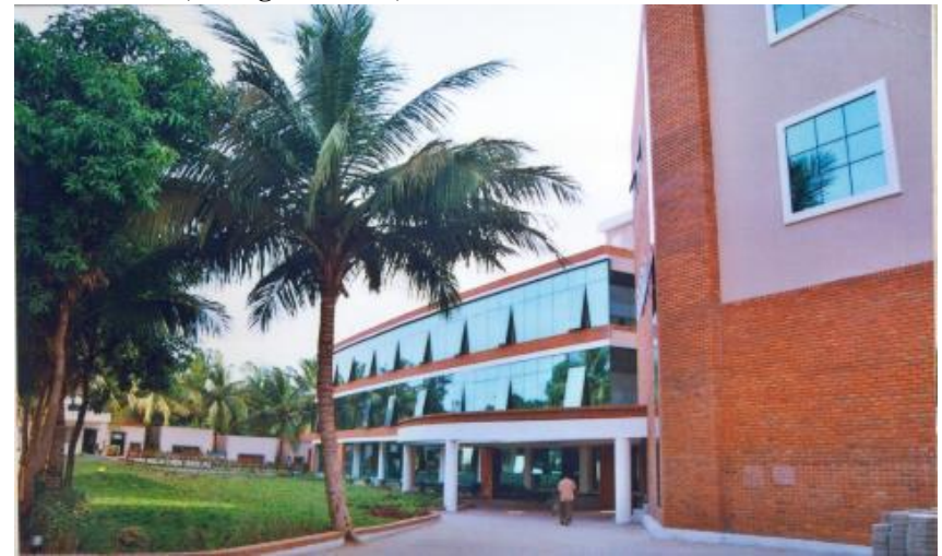
"Factory Building" for Ambattur Clothing Ltd, MEPZ, Chennai
