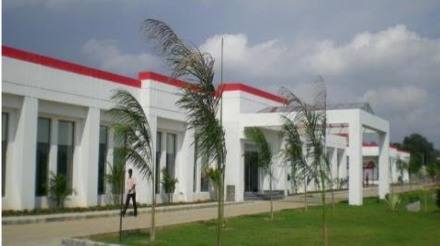
"Factory Building Project" for Triumph International India Pvt. Ltd, Singaperumal koil, Chennai
