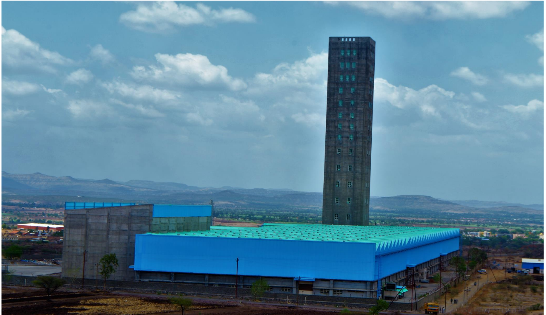
Factory Shed & VCV Tower for Finolex J- Power systems Private Ltd, Shirwal, Pune - 121 Meter height tall RCC structure
