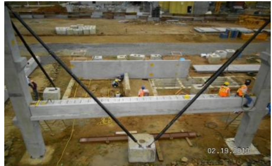
PRE. COLUMNS & INV. TEE BEAM IN POSITION
