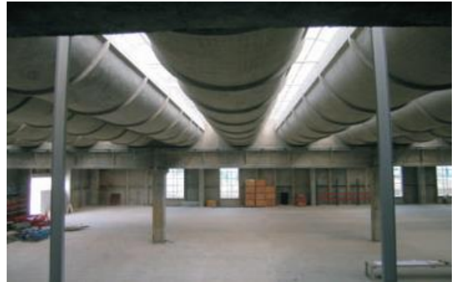
"Factory Building" for Rittal India Pvt. Ltd, Doddabalapur, Bangalore
