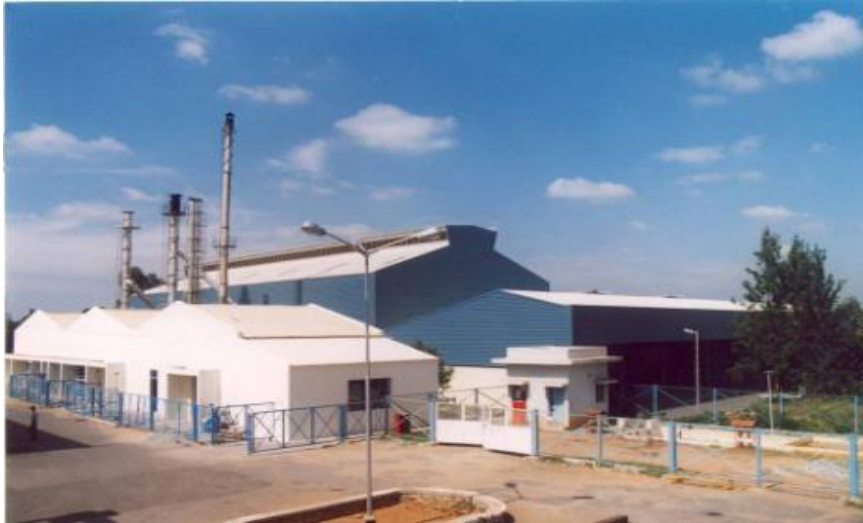
"Factory Building Extension" for Kirloskar Toyoda Textile Machinery Ltd, Jigini, Bangalore
