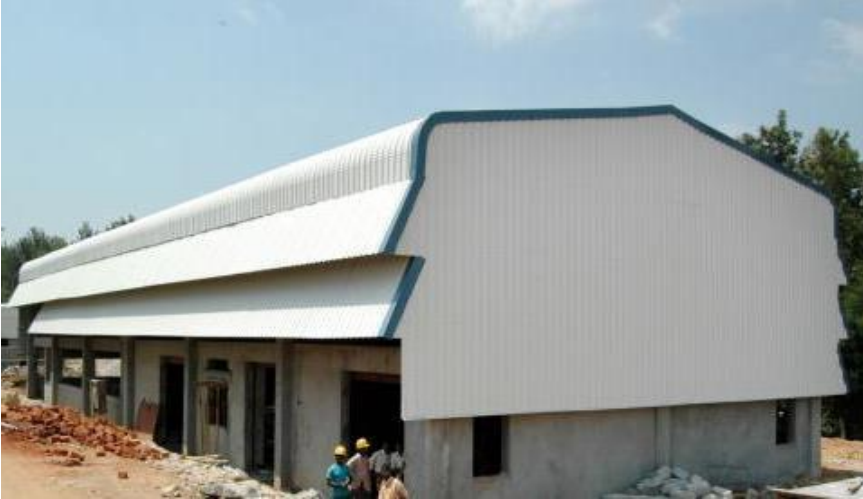
"Site Development & Road works" for ATC Beverages Ltd, Nanjangud, Mysore
