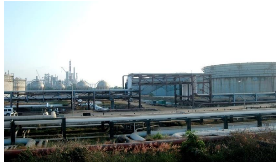
"MRPL - PFCC UNIT - (Phase - 3) Refinery Project" for Mangalore Refinery and petro chemical Ltd. Mangalore
