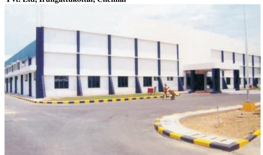
"Factory Building" for Mitsuba Sical (I) Ltd, Gummidipoondi, Chennai
