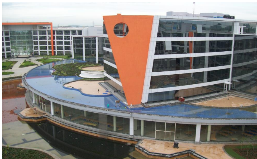
"Software Development Block (SDB- 5&6)" for Infosys Technologies Ltd, Mahindra World City, Chenglepet, Near Chennai
