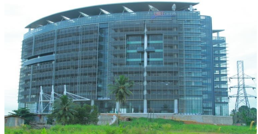
"IT Park" for UST Global Information Technology Parks Pvt Ltd, SEZ Campus, Attipra, Trivandrum
