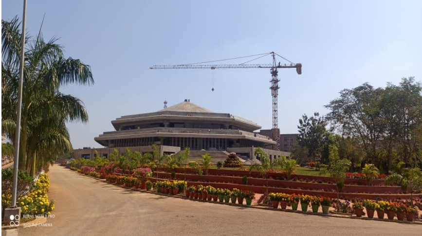
15000 Seating Capacity of Auditorium Building for Xavier University, Bhubaneswar, Odisha
