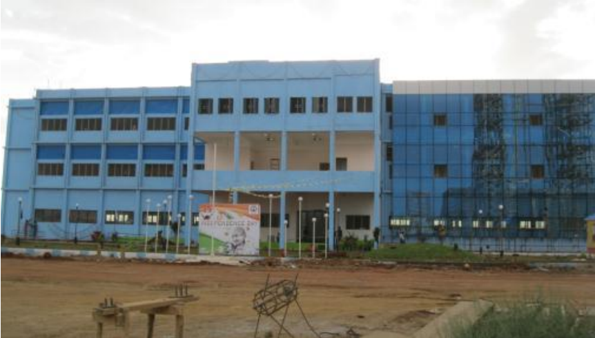
"2 X 500 MW Tuticorin Thermal Power project" for Bharat Heavy Electricals Ltd (BHEL),Tuticorin
