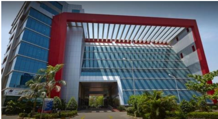
"BSNL Administration Office" for Bharat Sanchar Nigam Ltd (BSNL), Greams Road, Chennai
