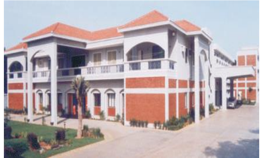
"Factory Building" for Twinkle Leatherwares India Ltd, Vandalur, Chennai
