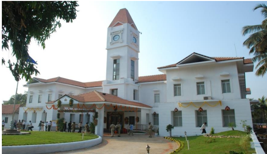
"New Commissionerate Building" for Karnataka State police housing corporation Ltd., DAR Compound Mangalore
