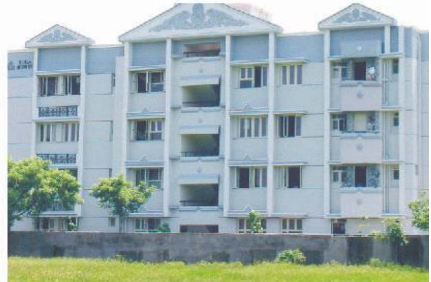
"Yuga Homes - Residential building" for Yuga Homes Ltd, Virugambakkam, Chennai
