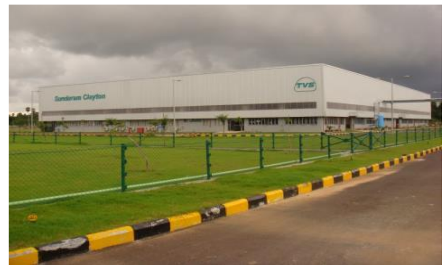
"Machine Plant" for TVS Sundaram Clayton Ltd, Mahindra World City, Chenglepet, Near Chennai
