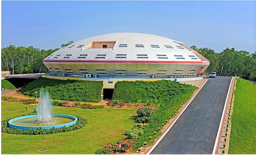
"Machine Control Center" for ISRO, Sulurpet
