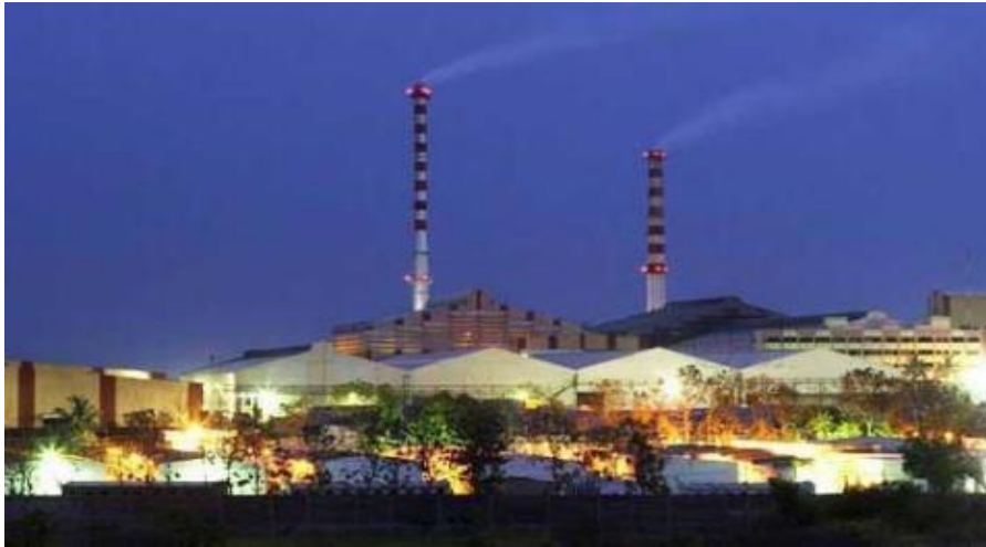
Glass Manufacturing Building for AGI Glaspac, Bhongir, Telangana
