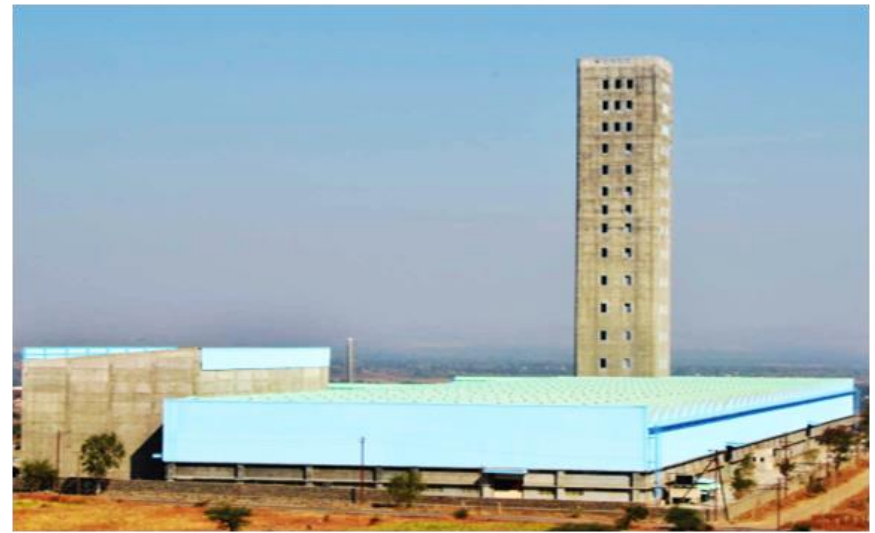
"Factory Shed & VCV Tower for EHVP cable project" for Finolex J-Power systems Private Ltd., Shirwal, Pune
