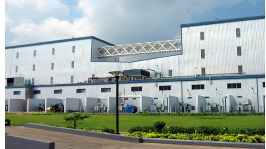
"Factory Building" for Apollo Tyres Pvt Ltd, Oragadam, Chennai
