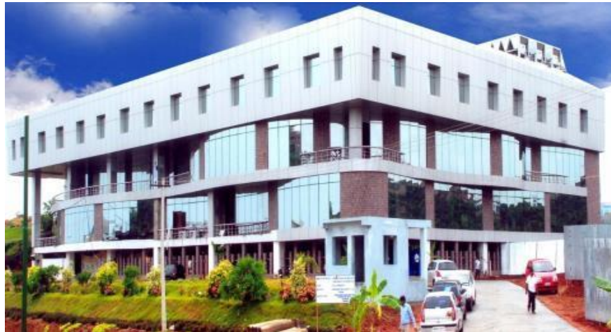
"Mahathi IT Park" for Mahathi Software Private Ltd, Madurawada, Vishakapatnam
