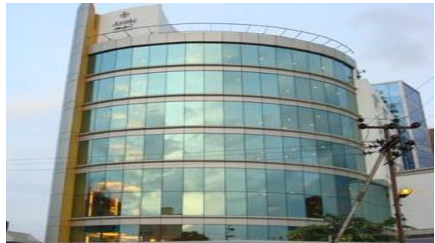
"Atithi Hotel" for Jayaram Hotels Pvt. Ltd, Kamaraj Salai, Puducherry – 2 Star 58 Rooms
