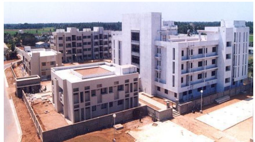
Staff Quarters, Nurses Hostel & Guest House for Aravind Eye Hospital & PG Institute of Ophthalmology, Puducherry
