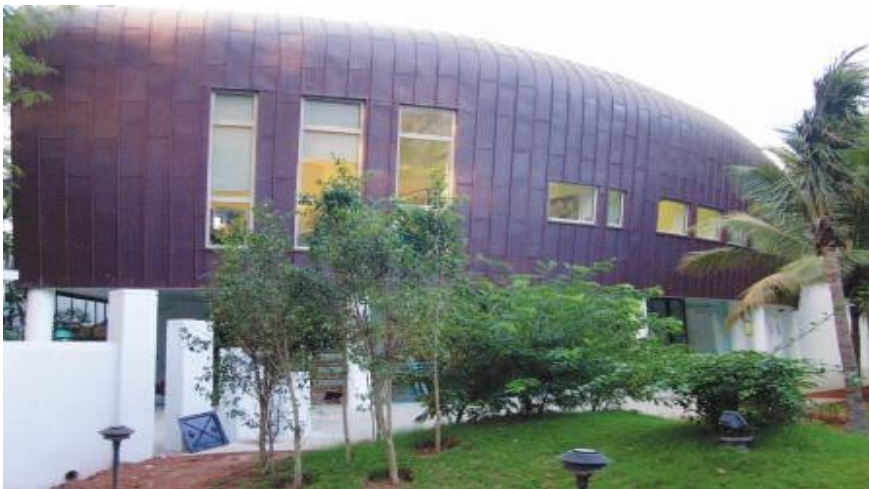
"Visa Office Building" for British Deputy High Commission (BDHC), Anderson Road, Chennai
