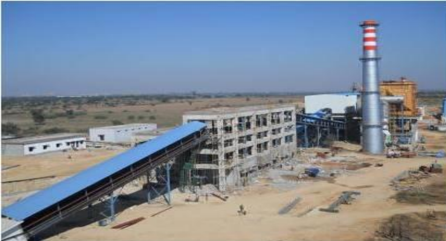
"Pellet plant-Factory Building" for XINDIA Steels Ltd. Kopal, Karnataka
