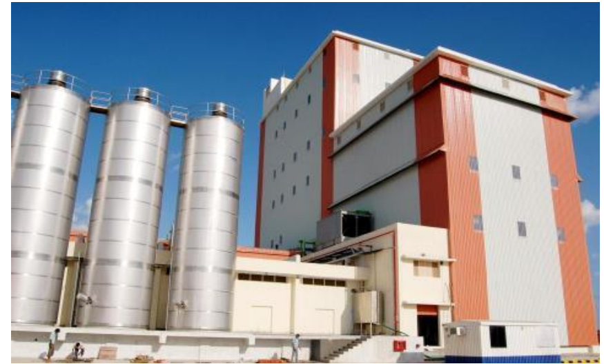
"Factory Building" for Hatsun Agro Product Ltd Krishnagiri
