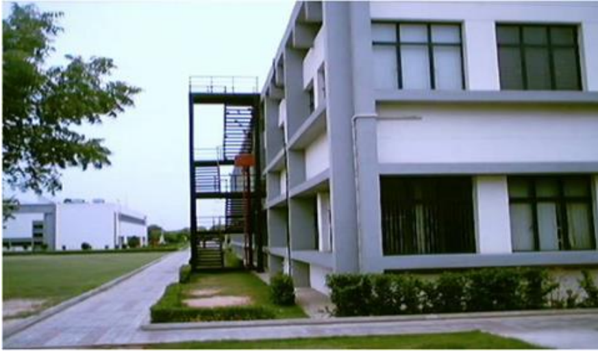
MICO Factory Building – PH 2 Precast for Motor industries Co Ltd, Sitapura, Jaipur
