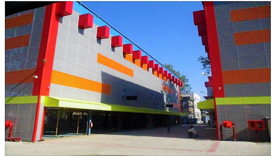
Fully Mechanized, Semi Automatic Multi Level Car Parking for Jammu & Kashmir Economic Reconstruction Agency Super Bazaar, Jammu - 352 Nos of 4 Wheeler & 164 Nos of 2 Wheeler
