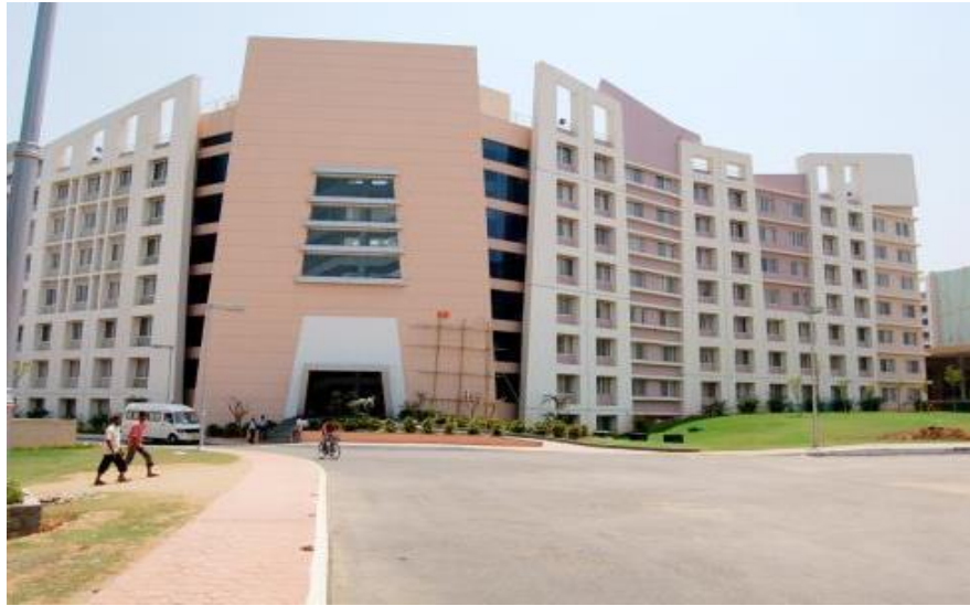
Infosys Hostel Building, Mysore, Karnataka
