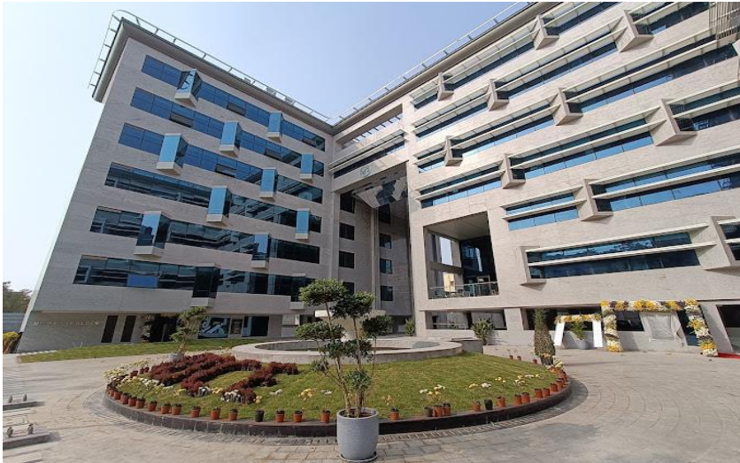
School Building for Council for the Indian School Certificate Examinations , Hyderabad
