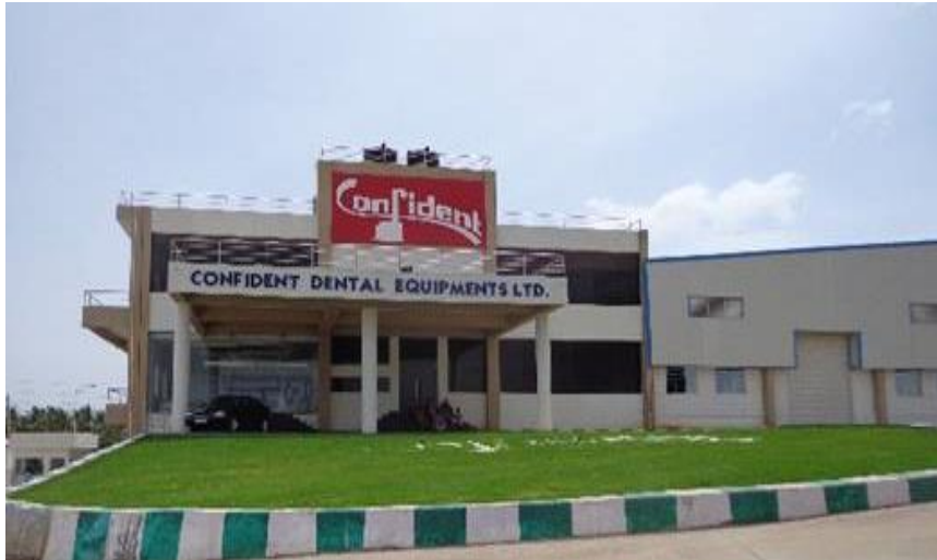
"Factory Building" for Confident Dental Equipment, Bidadi Industrial Area, Bangalore
