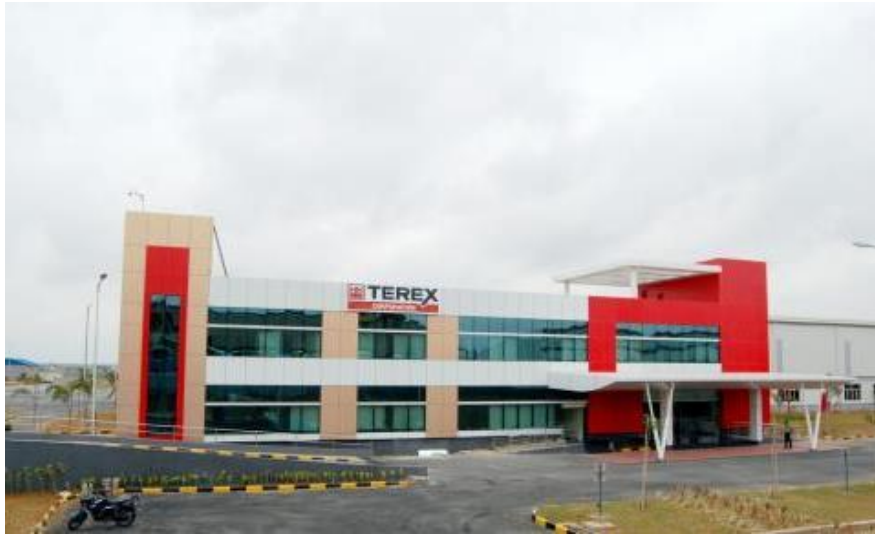
"Land Development Retaining Wall and Compound Wall" for Terex India Ltd, SIPCOT Industrial Area (Phase II), Hosur
