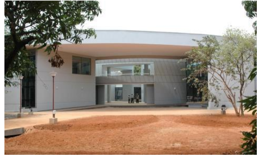
Factory Building for Hindustan Lever Ltd, HLRC, White Field, Bangalore
