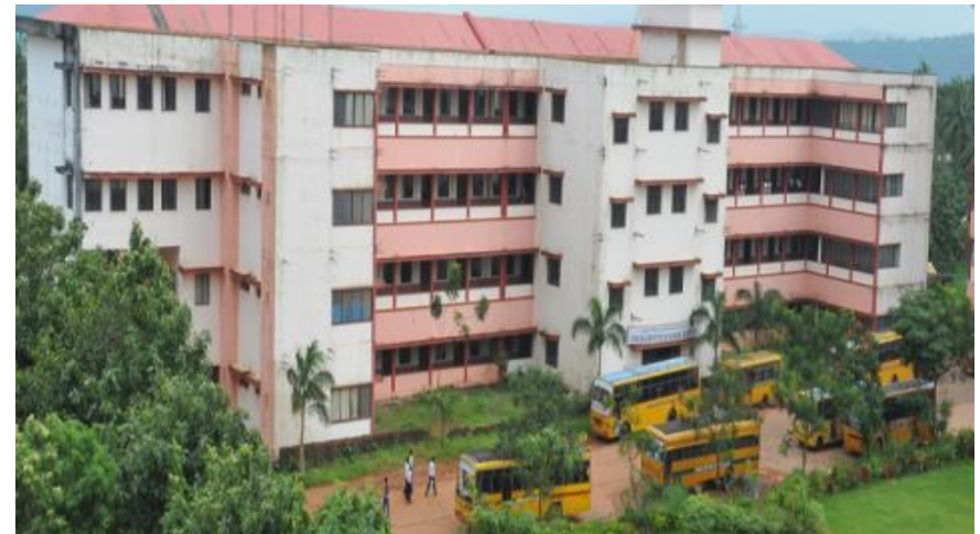
Dental College Building & Hostel for A Shama Rao Foundation, Mukka Campus, Karnataka
