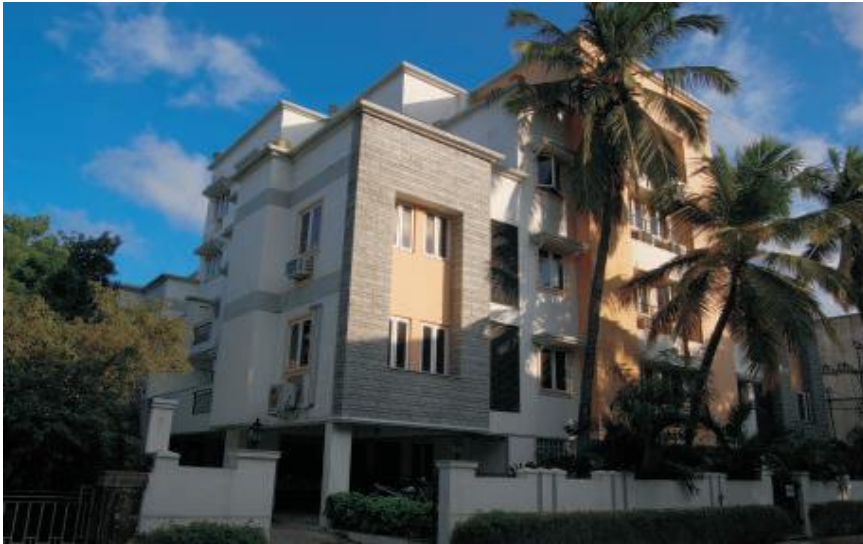
"Mithila - Residential Building" for Yuga Homes Ltd, Mylapore, Chennai
