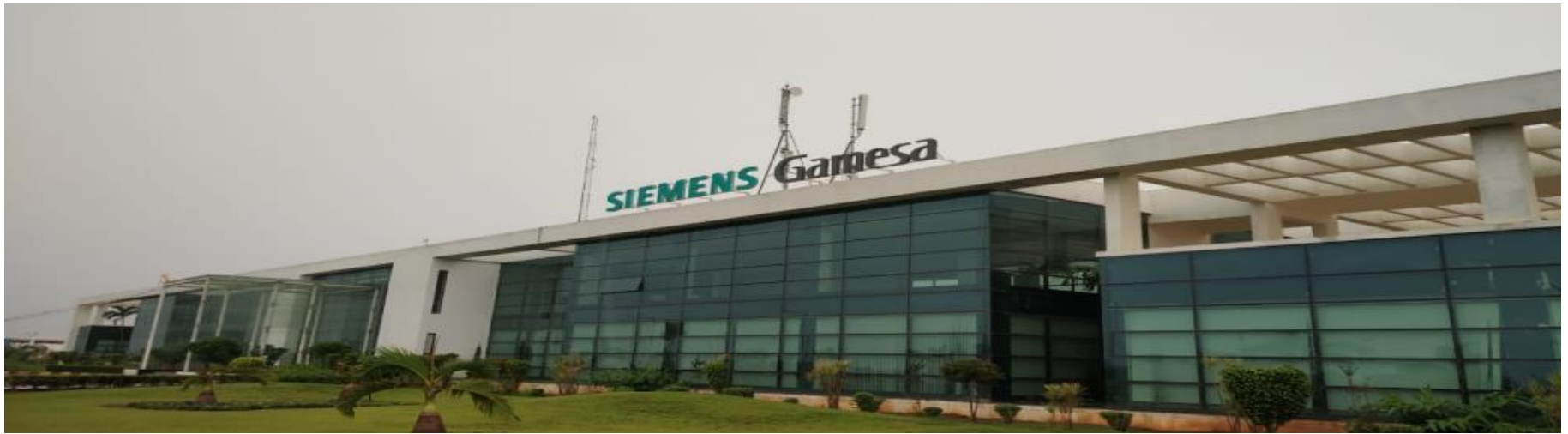
Admin Building & Warehouse Building for Gamesa Renewable Private Limited, SPSR Nellore, Andhra Pradesh
