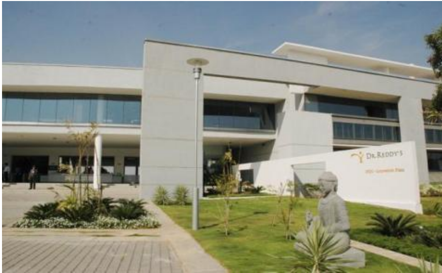
Construction of IPDO Center for Dr.Reddy's Laboratories Ltd, Bachuppalli, Andhra Pradesh
