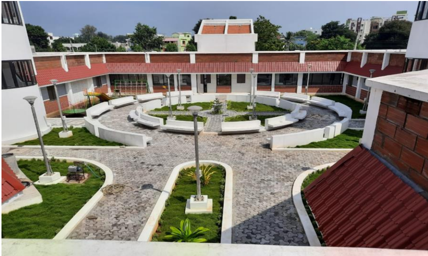
The Salvation Army Evangeline Booth Hospital Nidubrolu, Andhra Pradesh – 50 Beds
