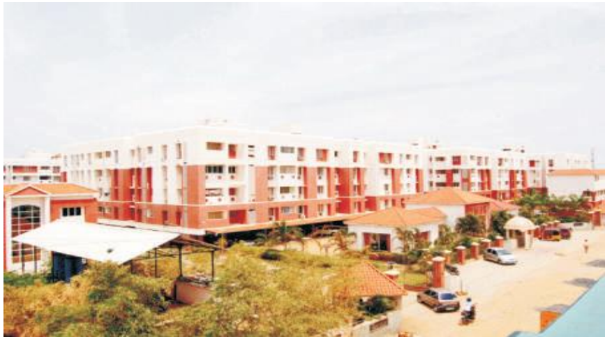
"Residential Building" for True Value Homes India Pvt Ltd, Thoraipakkam, Chennai
