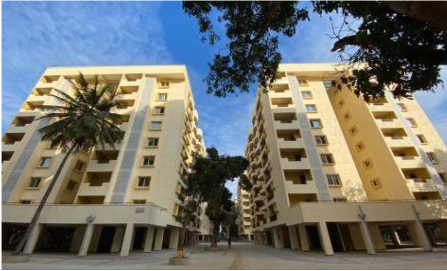
Residential Quarters for Bharat Electronics Ltd , BE Estate, Bangalore
