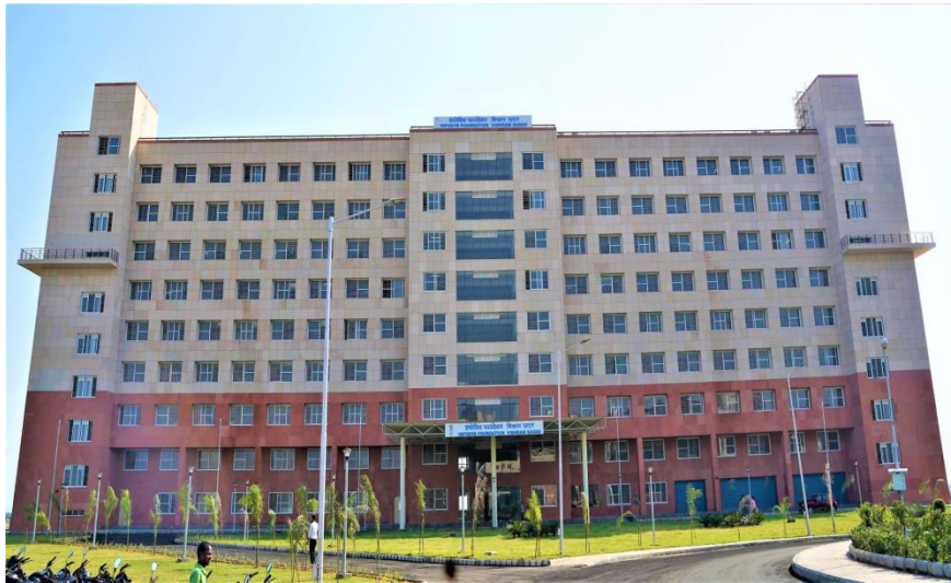
Vishram Sadan for Infosys Foundation at National Cancer Institute (NCI) Campus of AIIMS, Jhajjar, Haryana – 806 Beds
