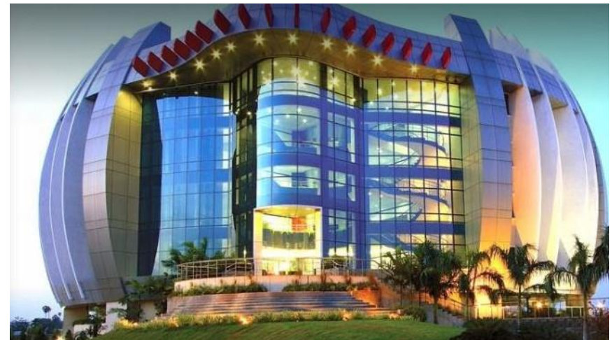
"KRISP IT Park - IT Building" for Krishnan Sivagami Pvt Trust, Kizhakottaiyur, Chennai
