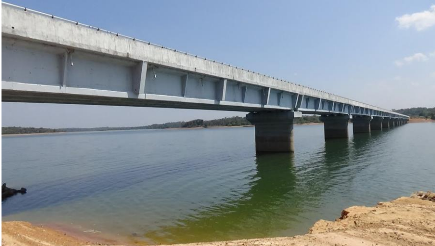
Sagar - Pattaguppa Road Shimoga Bridge for Karnataka Road Development Corporation Ltd , Hasanagar Taluk, Shimoga District, Karnataka.
