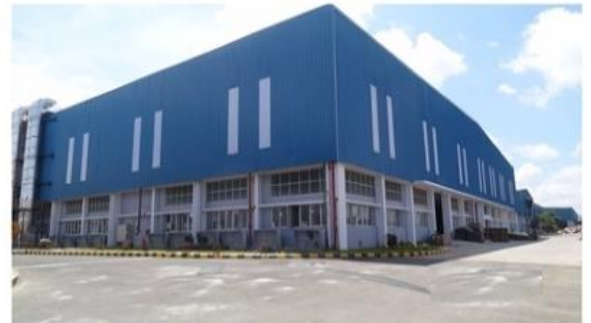
"Block III Building-Manufacturing Phase" for Flowserve Inida Controls Pvt Ltd, Myleripalayam post, Coimbatore
