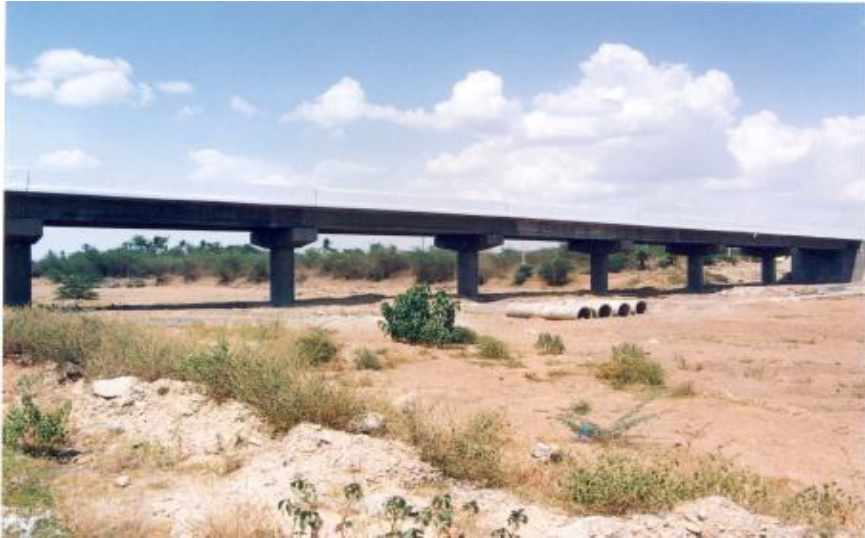
"Polur Bridge" for Highways Department, Polur, Tiruvannamalai,
