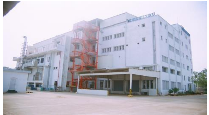
Press Building for Kasturi & Sons Limited The Hindu for , Maraimalai nagar, Chengalpet, T.N
