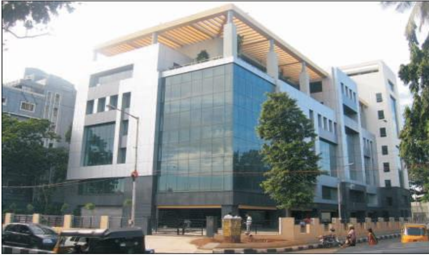
"Mr.R.Ramanathan's Office Building", Chetpet, Chennai
